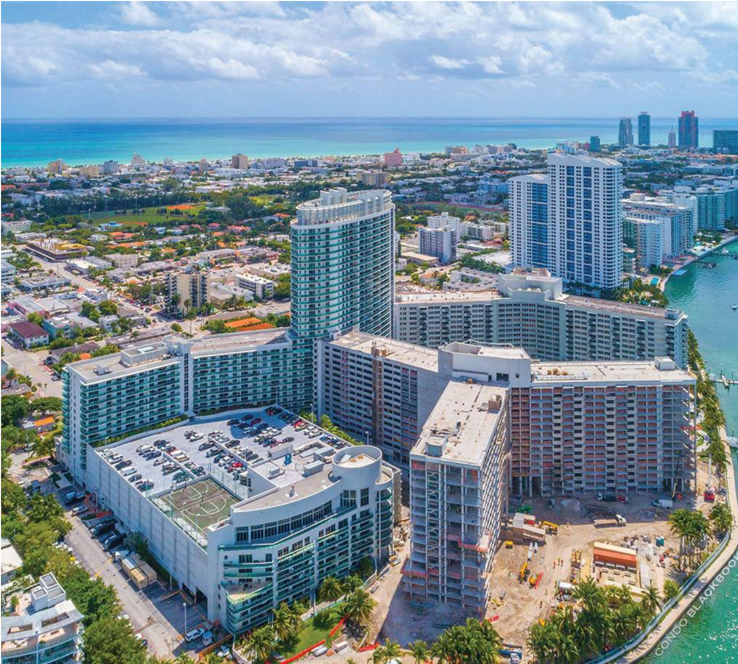
Existing Penthouse Aerial View
