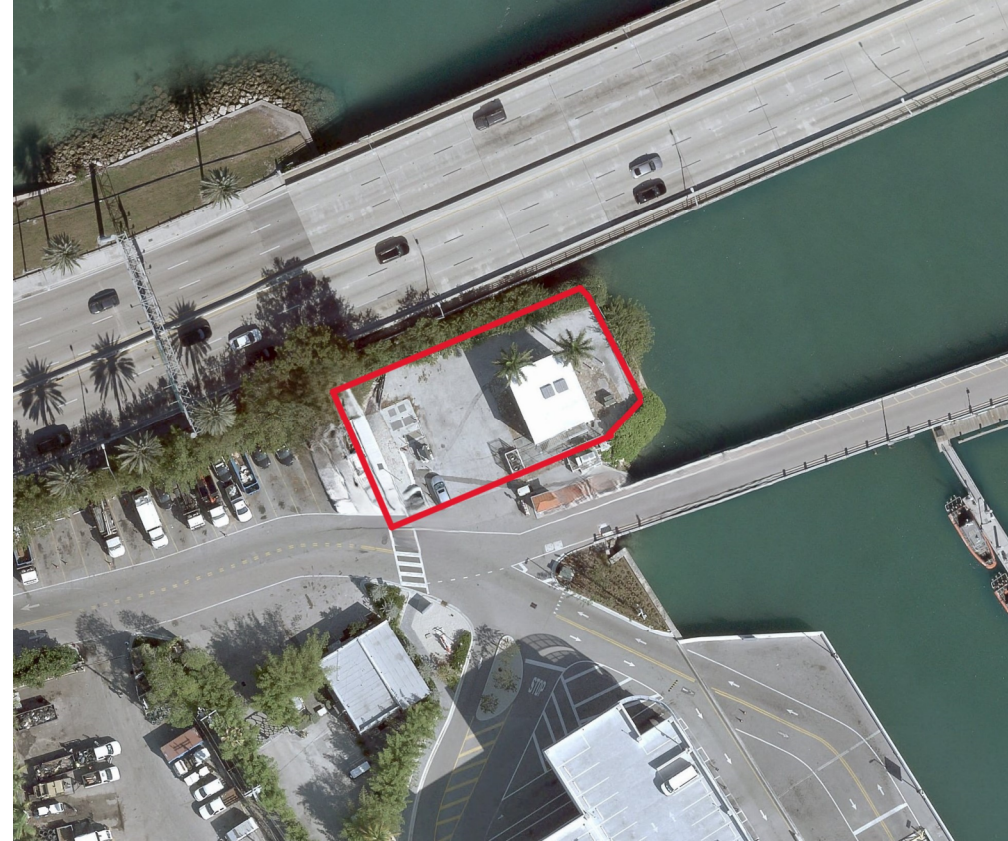
TERMINAL ISLAND WATER BOOSTER PUMP STATION HARDENING
