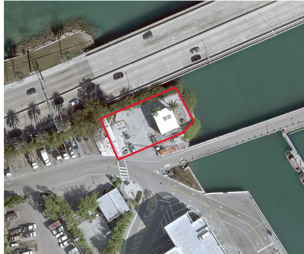
TERMINAL ISLAND WATER BOOSTER PUMP STATION HARDENING
