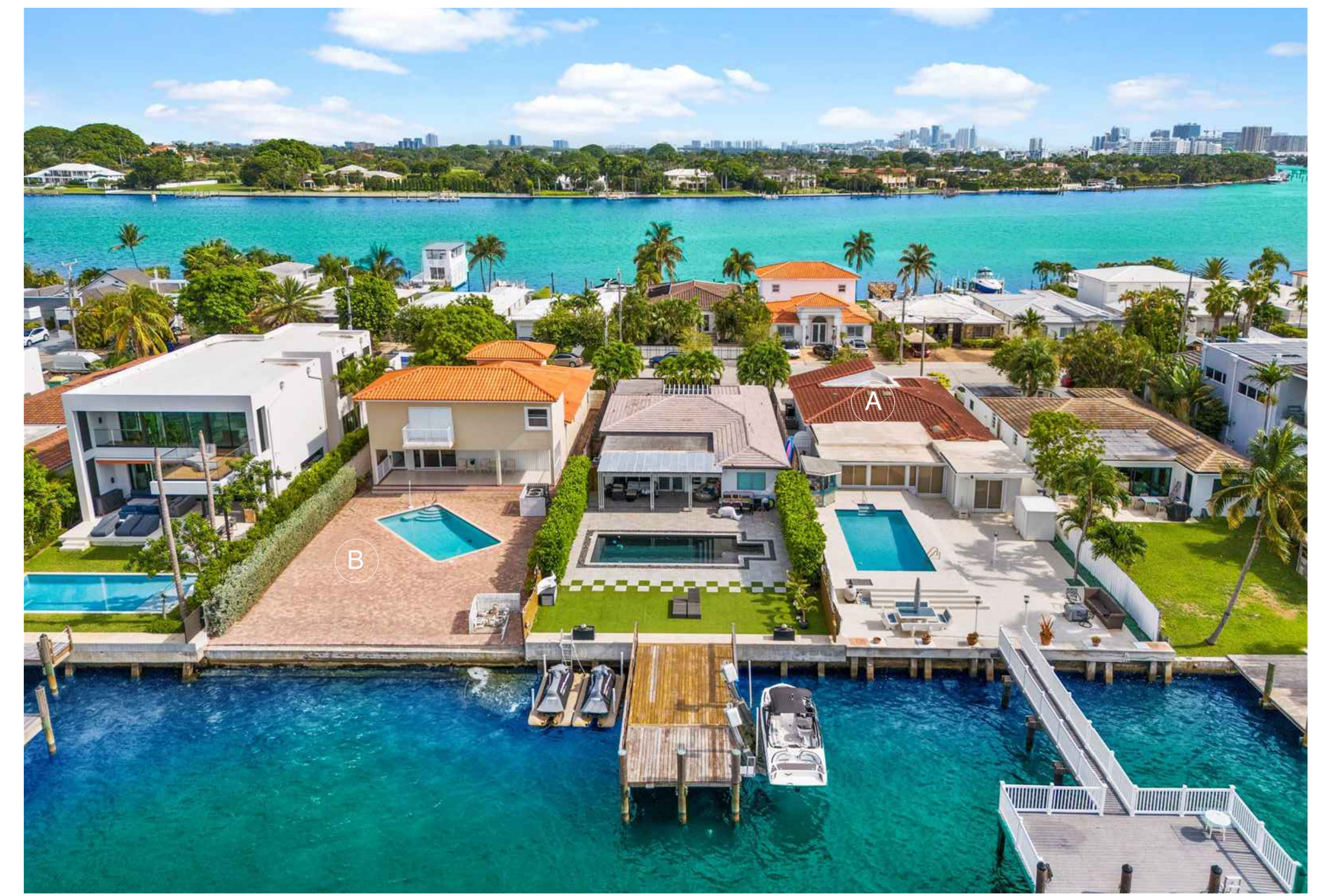
02 NEIGHBORING PROPERTIES EAST AND WEST (REAR VIEW) SCALE: N/A
