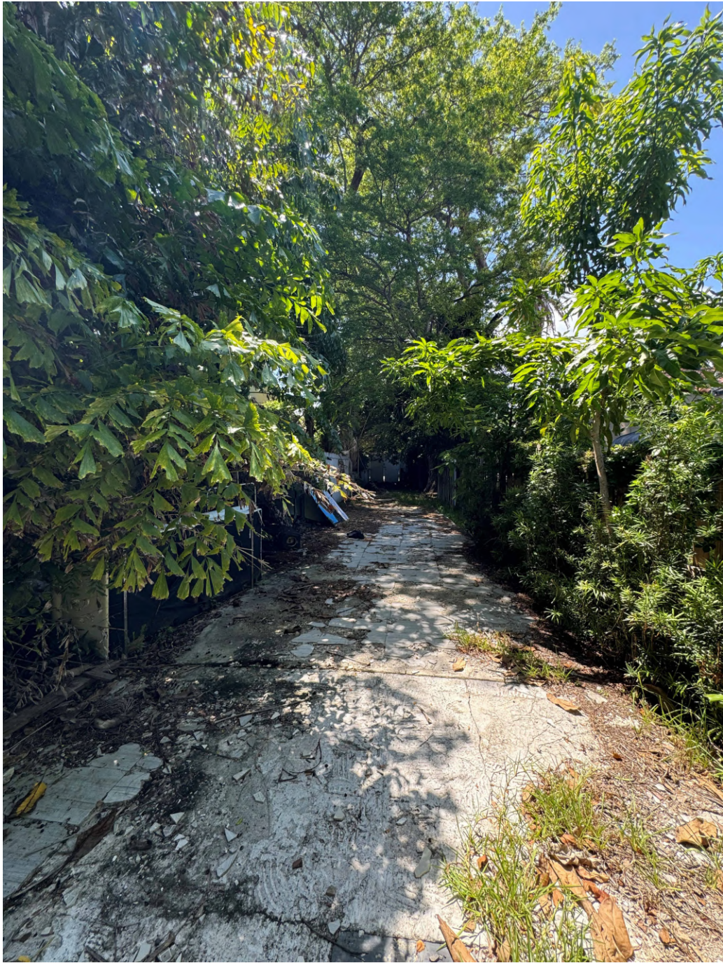
6. EXISTING INTERIOR CONDITION PROJECT SITE
