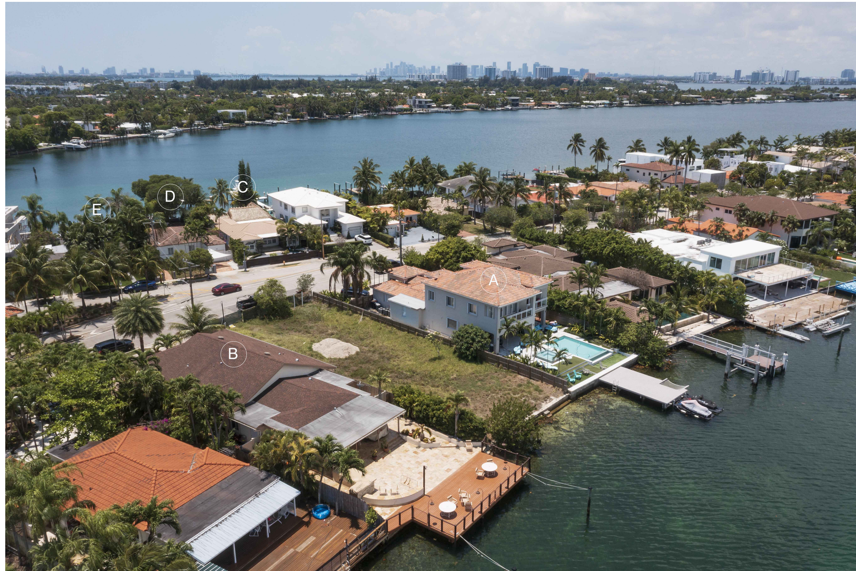
03 NEIGHBORING PROPERTIES (AERIAL VIEW) SCALE: N/A
