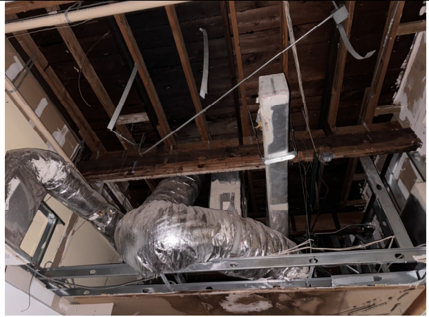
Photo 8 – Interior partitions in poor conditions, presence of humidity due to lack of waterproofing in the roof.
