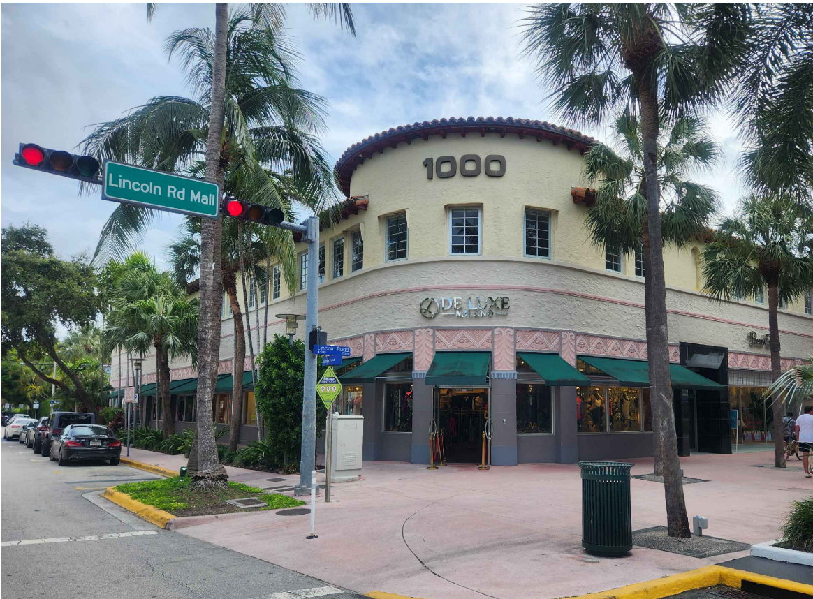
A1 SOUTH-WEST CORNER INTERCEPTION OF LINCOLN ROAD AND MICHIGAN AVE PHOTO TAKEN: 06-12-2024
