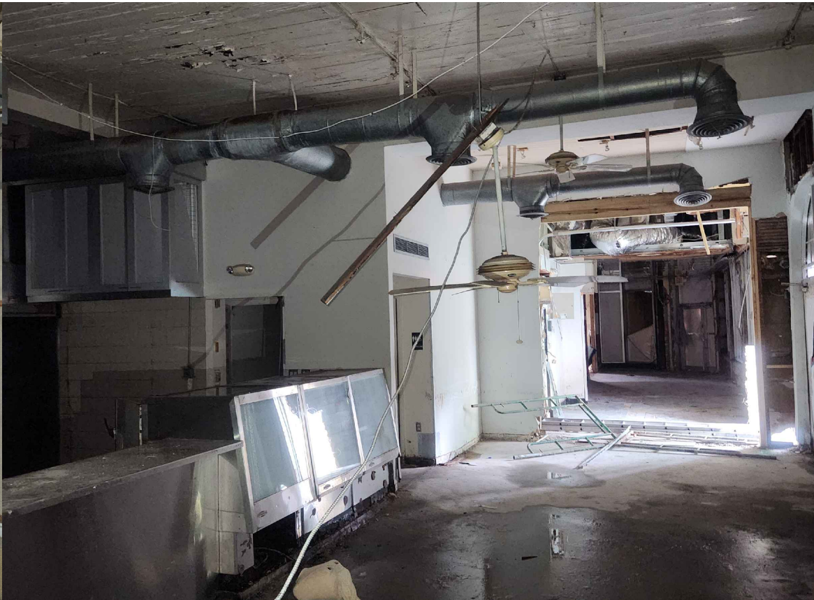
C4 CURRENT EXISTING INTERIOR OF THE BUILDING: VIEW THROUGH DIFFERENT LOCALS PHOTO TAKEN: 06-12-2024
