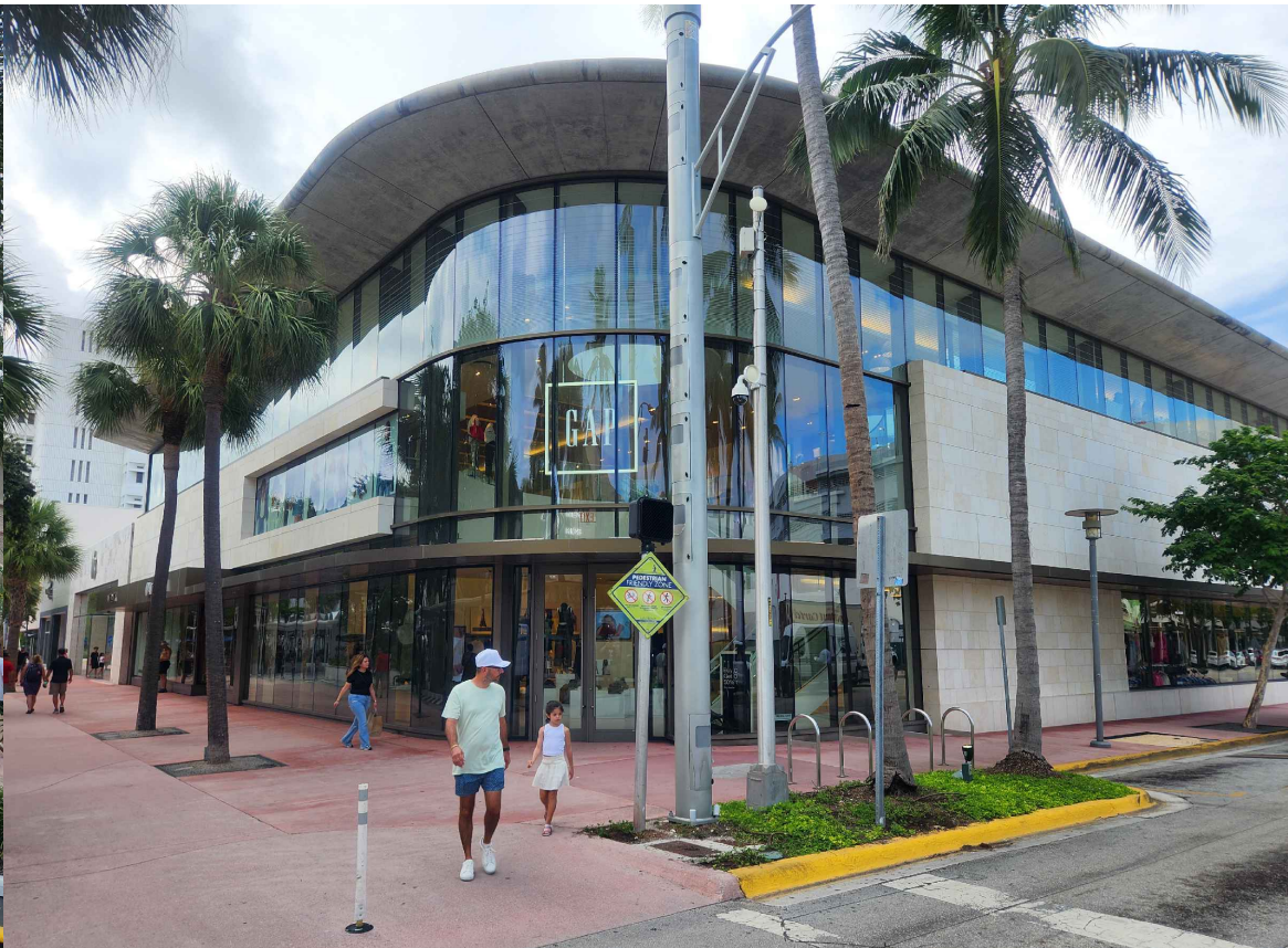
A4 NORTH-WEST CORNER INTERCEPTION OF LINCOLN ROAD AND MICHIGAN AVE PHOTO TAKEN: 06-12-2024
