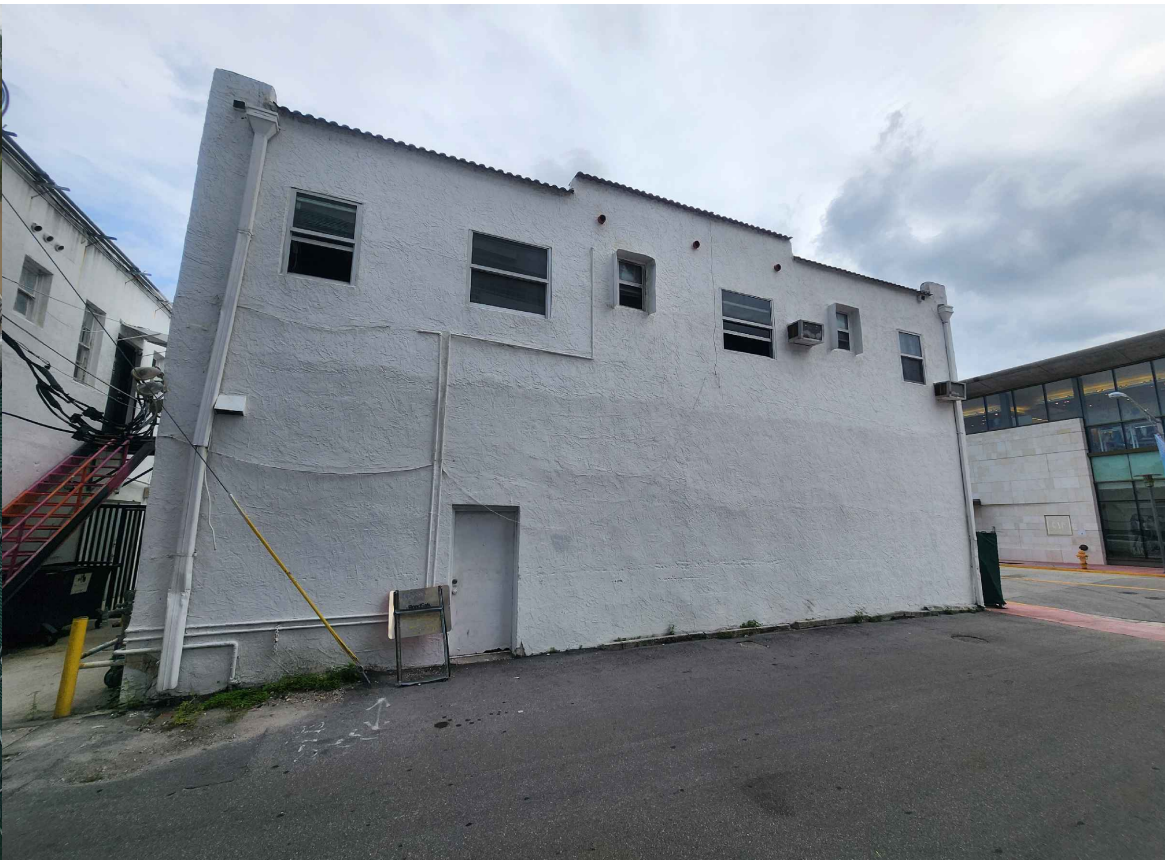
A4 NORTHERN BUILDING FACADE @ LINCOLN LN. N PHOTO TAKEN: 06-12-2024
