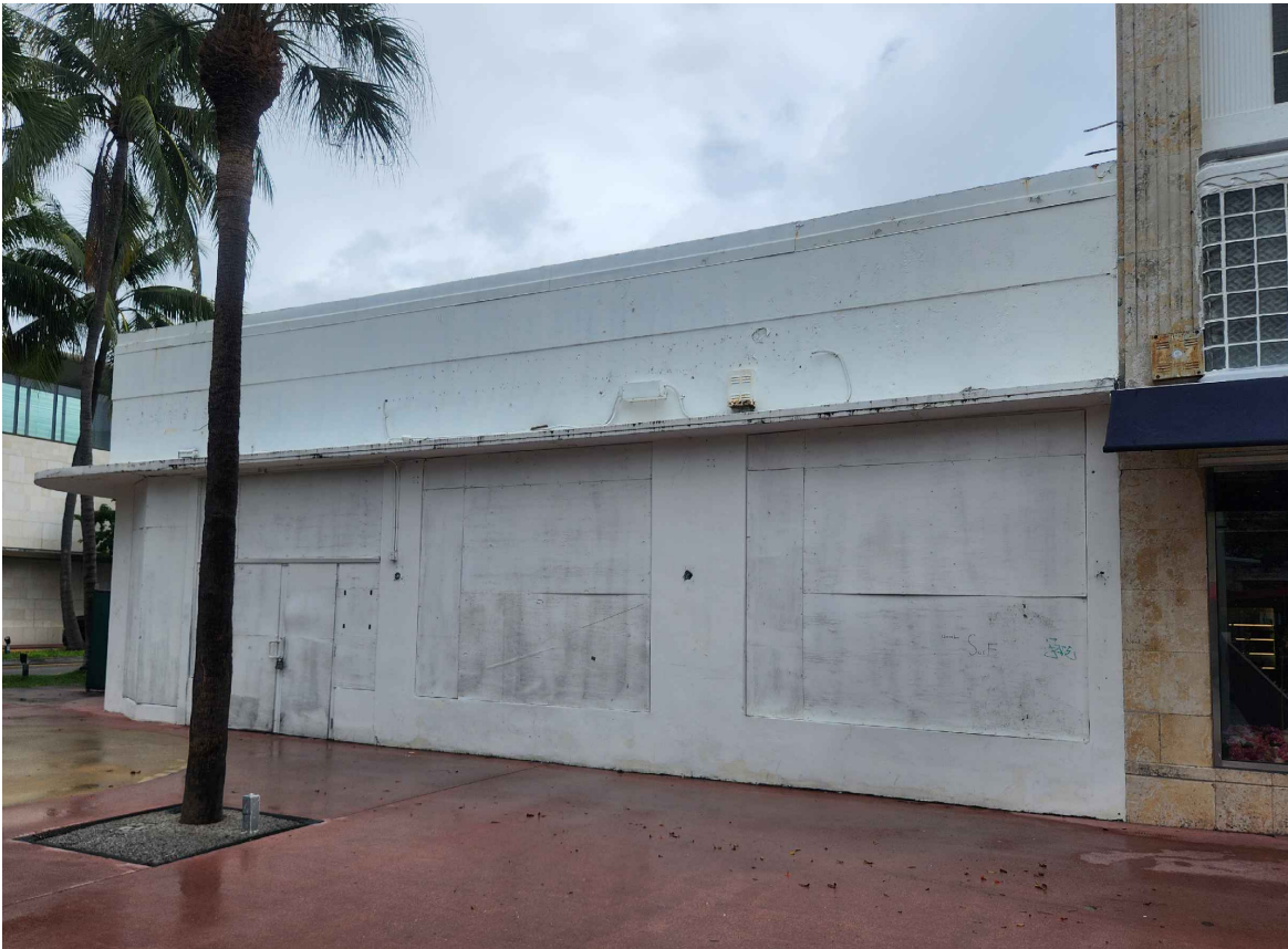
C1 SOUTHERN BUILDING FACADE (FRONTAGE AT LINCOLN ROAD) PHOTO TAKEN: 06-12-2024
