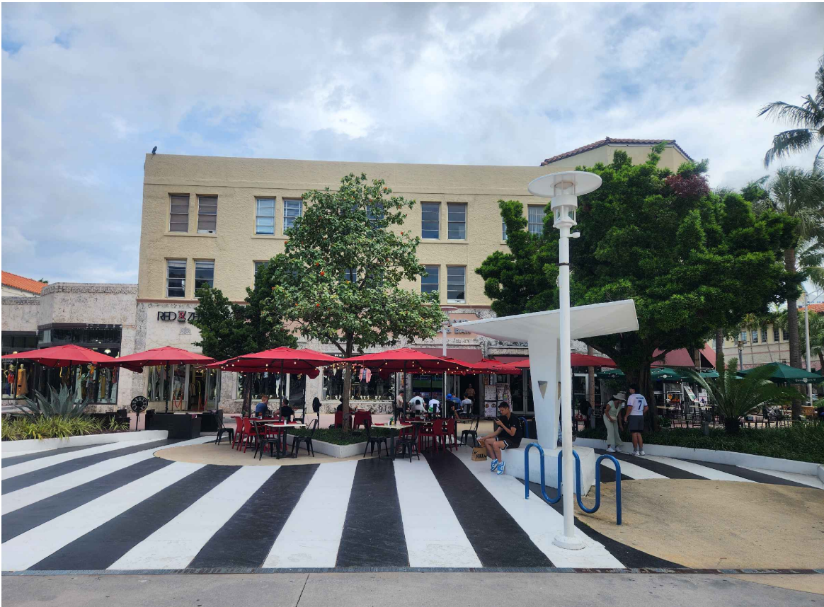
C1 ADJACENT BUILDING FRONTING 947 BUILDING @ LINCOLN ROAD PHOTO TAKEN: 06-12-2024
