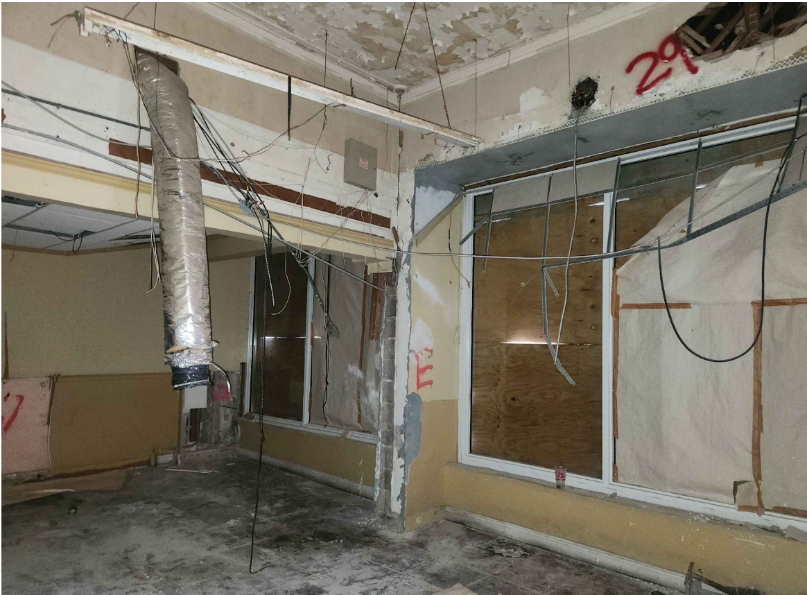
C1 CURRENT EXISTING INTERIOR OF THE BUILDING: VIEW THROUGH DIFFERENT LOCALS PHOTO TAKEN: 06-12-2024
