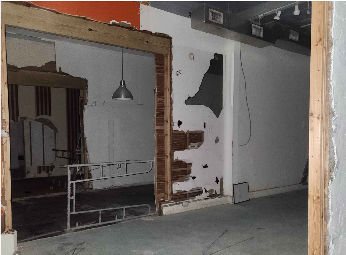
A1 CURRENT EXISTING INTERIOR OF THE BUILDING: VIEW THROUGH DIFFERENT LOCALS PHOTO TAKEN: 06-12-2024
