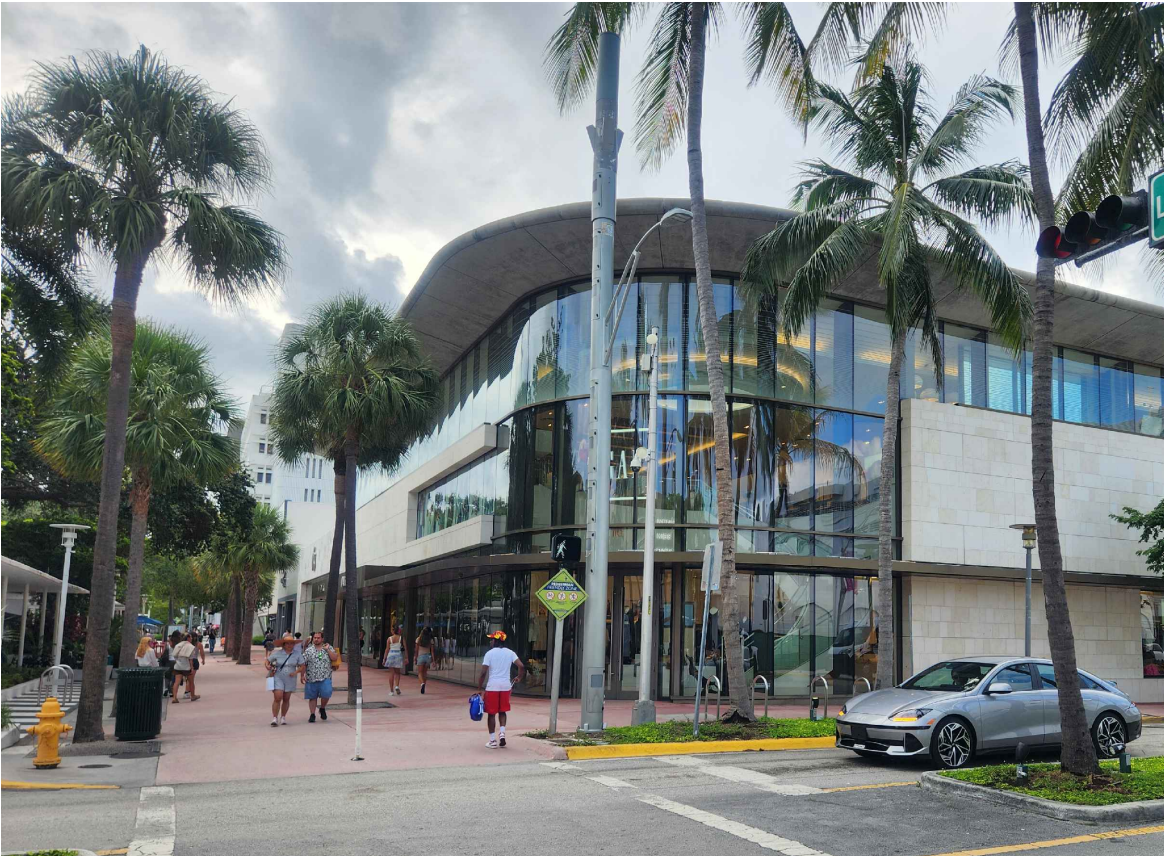
A1 NORTH-WEST CORNER INTERCEPTION OF LINCOLN ROAD AND MICHIGAN AVE PHOTO TAKEN: 06-12-2024
