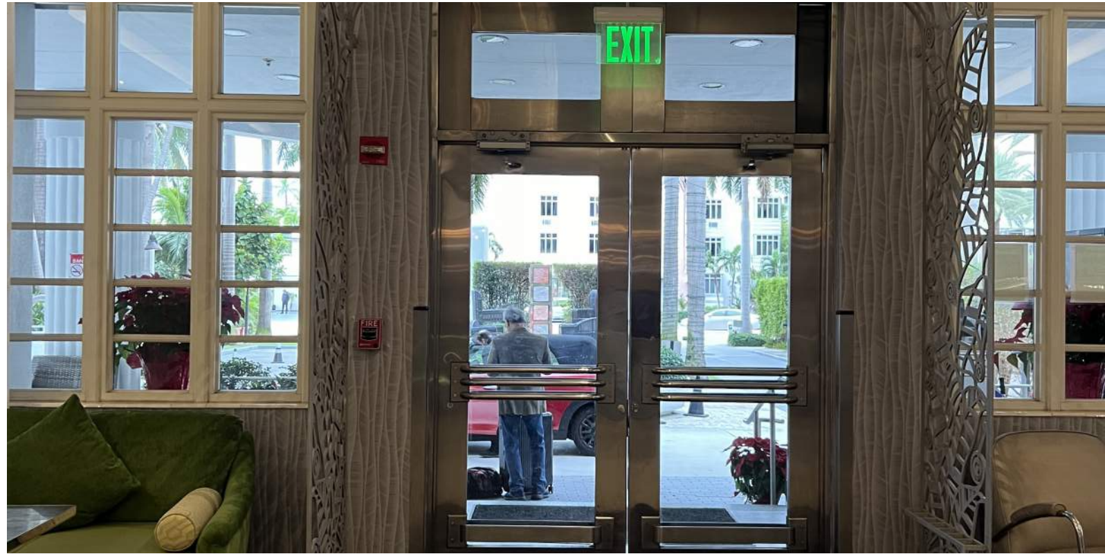
ENTRY FROM INTERIOR OF LOBBY
