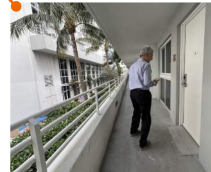
LANAI BUILDING EXTERIOR CORRIDOR
