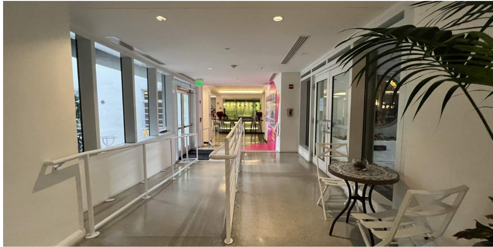
RAMP TO LOBBY
