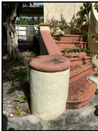
MAIN EXTERIOR STAIRS
