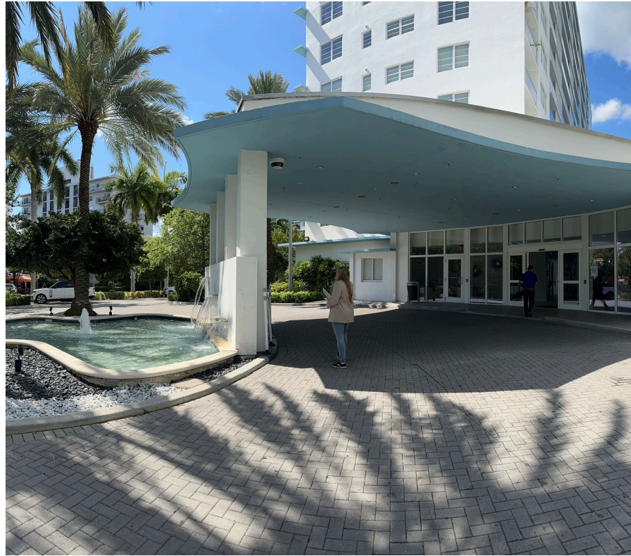
Existing Entry Canopy and Fountain
