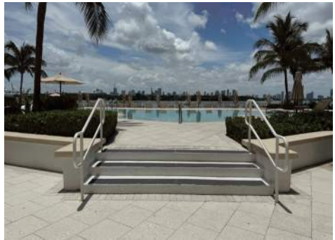
Existing Guardrail & Pool Pavers to match at the New Stairs
