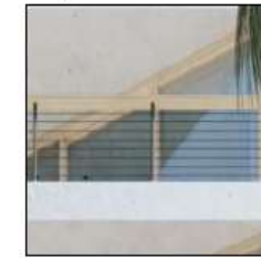
④ HORIZONTAL WIRE RAILING DETAIL
