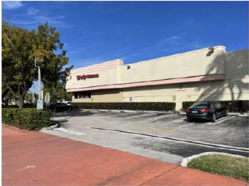
22 ALTON ROAD LOOKING NORTH EAST AT WALGREENS
