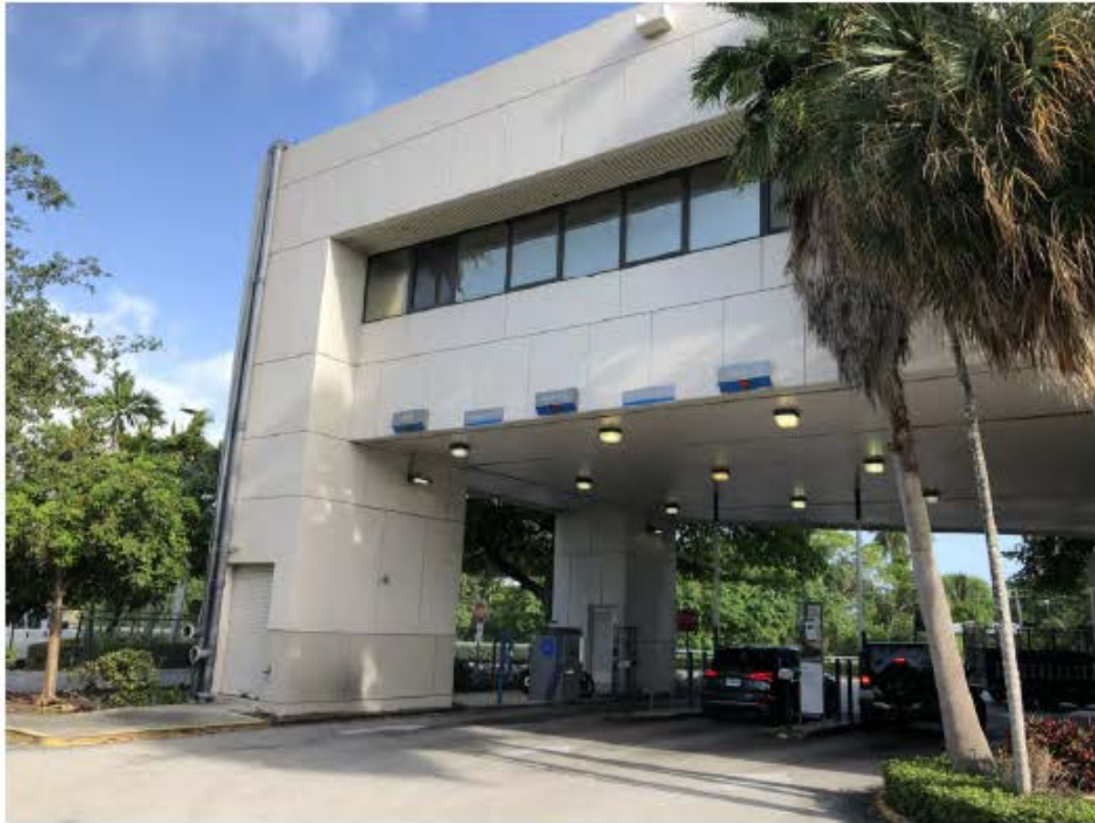
11 EXISTING PARKING LOOKING SOUTHEAST
