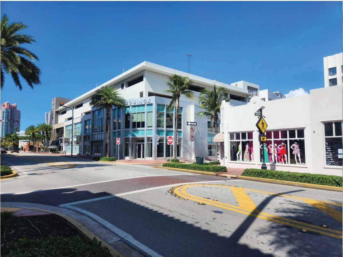
C1 VIEW FROM WESTERN SIDEWALK ON COLLINS AVE. @ THE INTERCEPTION OF COLLINS AVE. AND 6TH STREET PHOTO TAKEN: 06-20-2023
