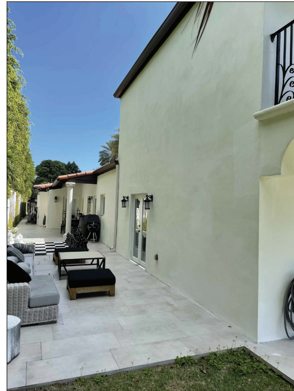
E2 - 6470 ALLISON RD - VIEW TO NORTH SIDE (EXISTING STRUCTURE)
