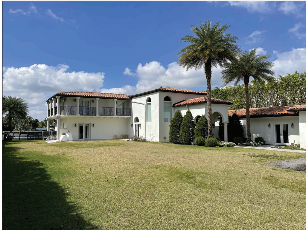
E3 - 6470 ALLISON RD - VIEW TO SOUTH SIDE (EXISTING STRUCTURE)
