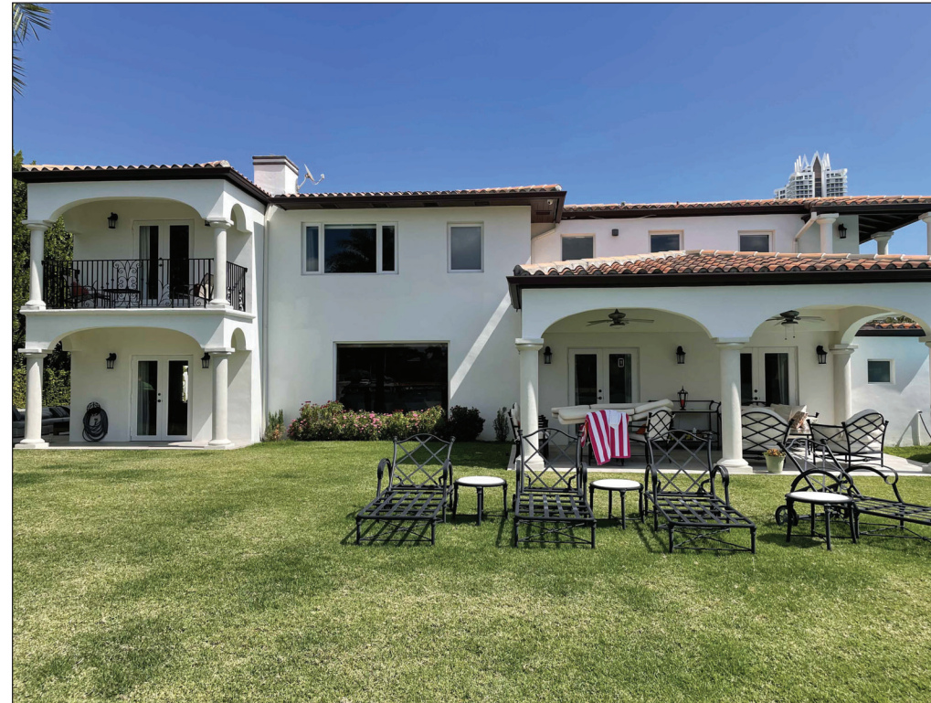
E4 - 6470 ALLISON RD - VIEW TO REAR (EXISTING STRUCTURE)
