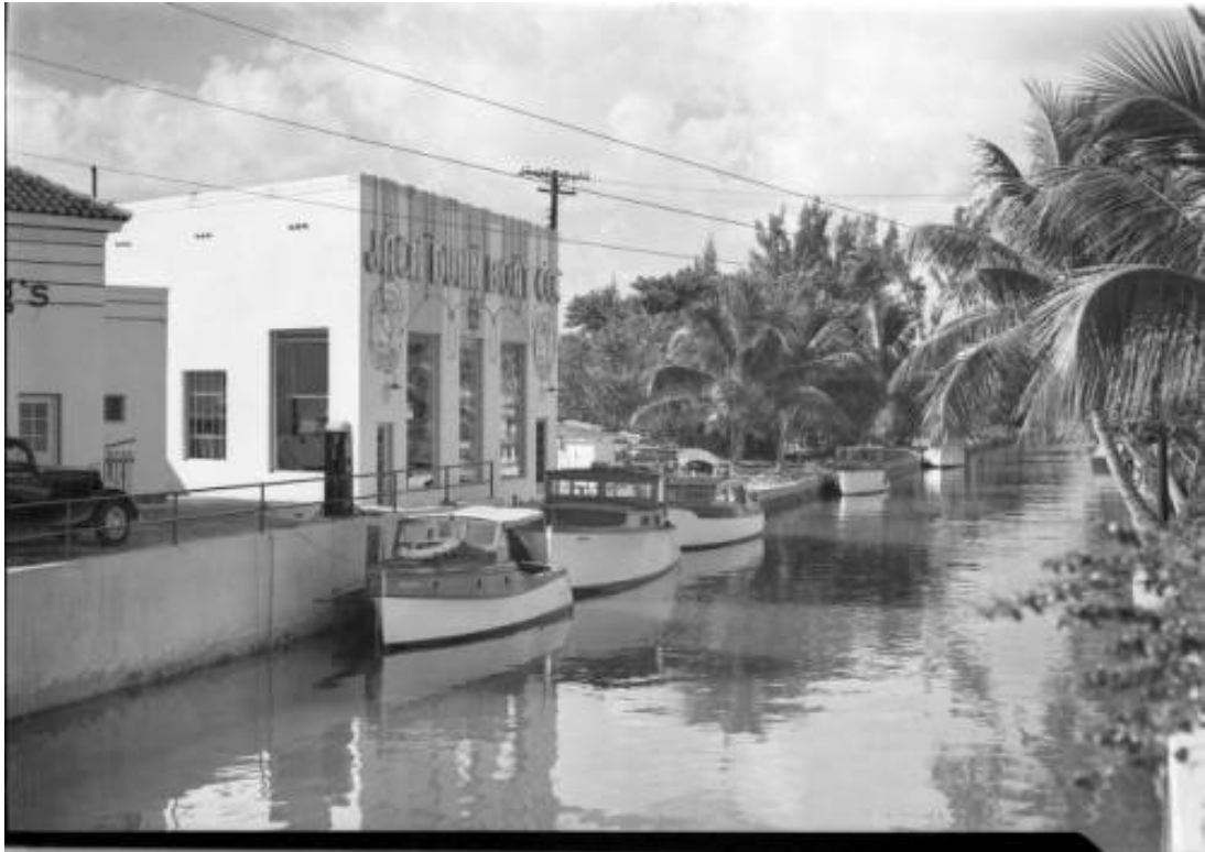
Photograph of Jack Dunn Boat Company (1740 Alton Road) and Collins Canal, 1938
