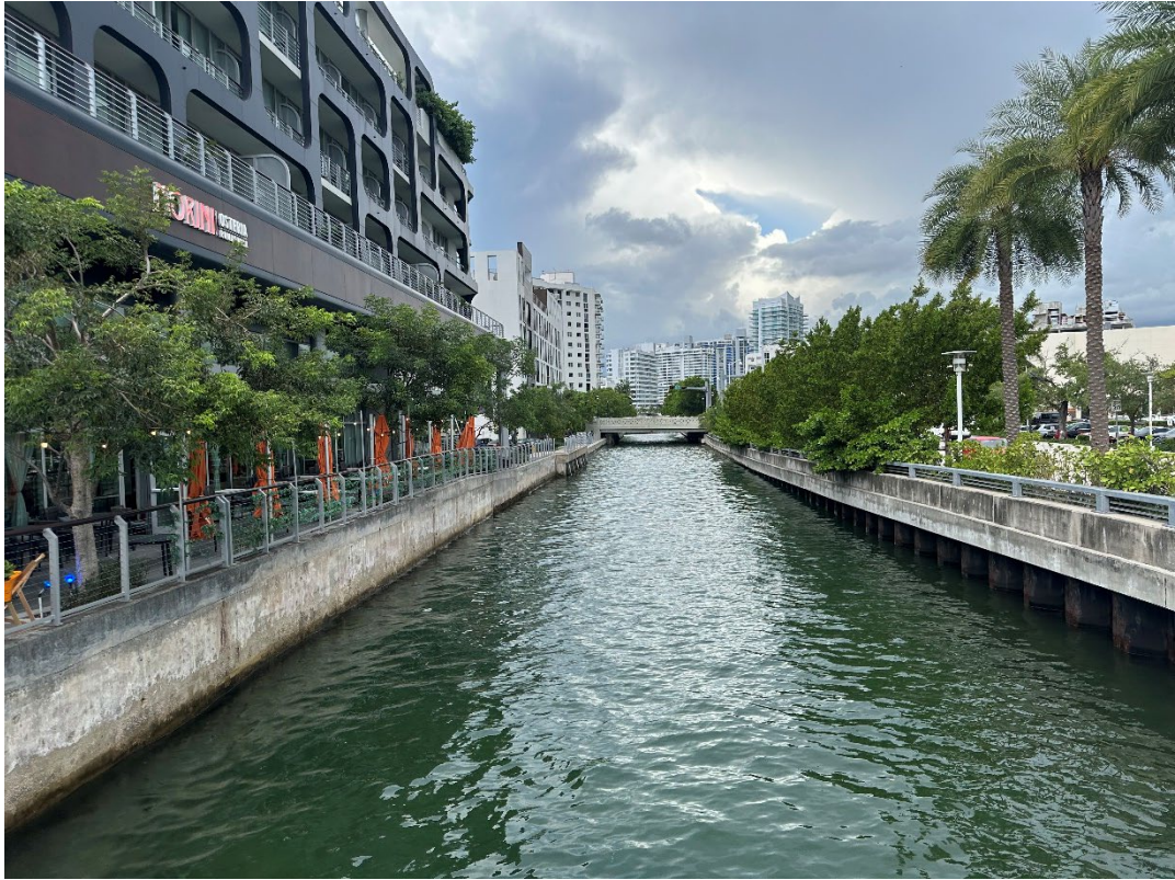
Collins Canal at Alton Road (looking west)
