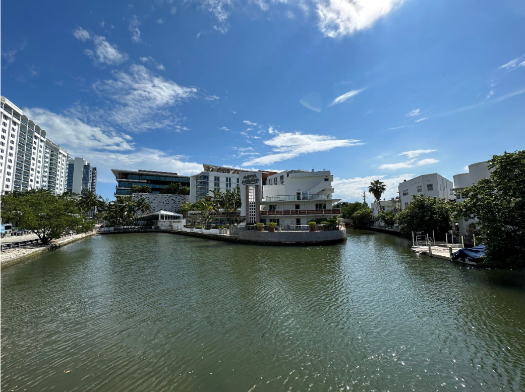
Collins Canal (right) at Lake Pancoast Pedestrian Bridge (looking east)
