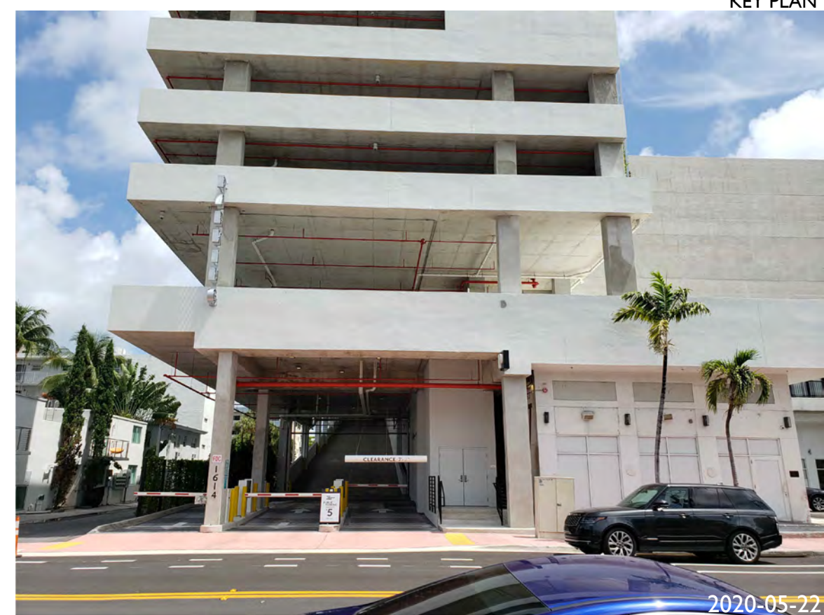
6. 1212 LINCOLN ROAD BUILDING - ENTRANCE TO GARAGE
