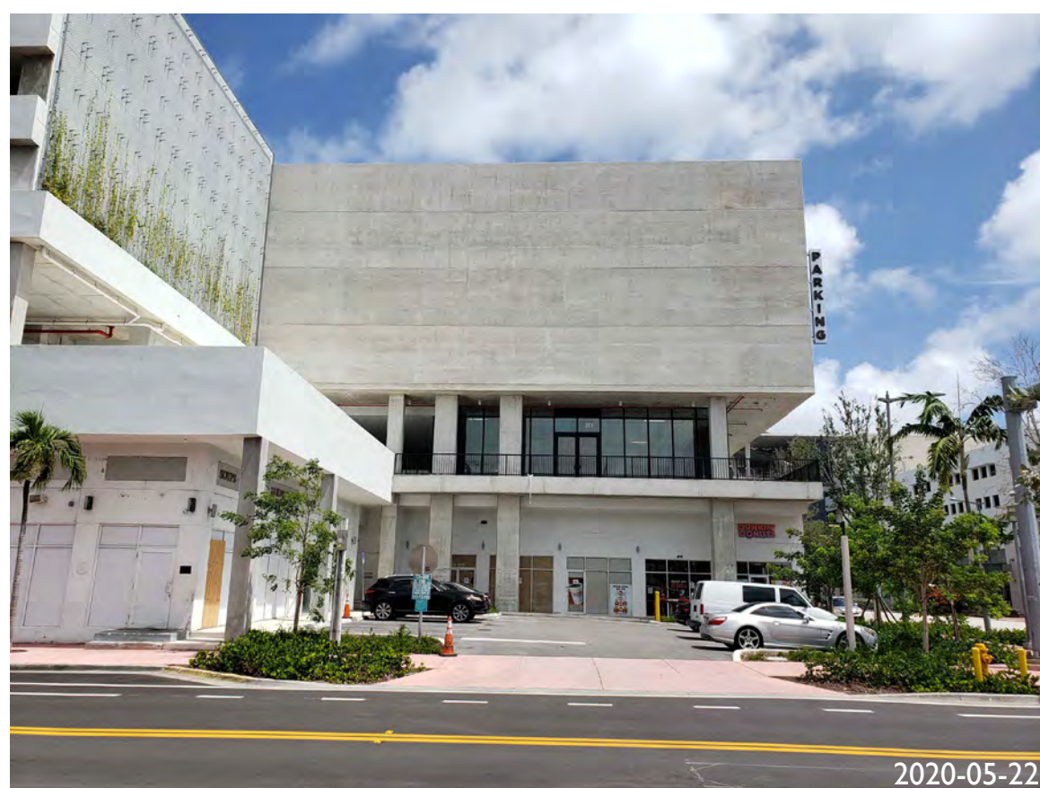
5. 1212 LINCOLN ROAD BUILDING - SOUTH PORTION
