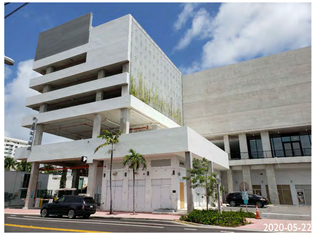
7. 1212 LINCOLN ROAD BUILDING - SOUTHEAST
