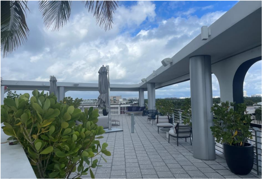
2 ROOF TERRACE / NORTH
