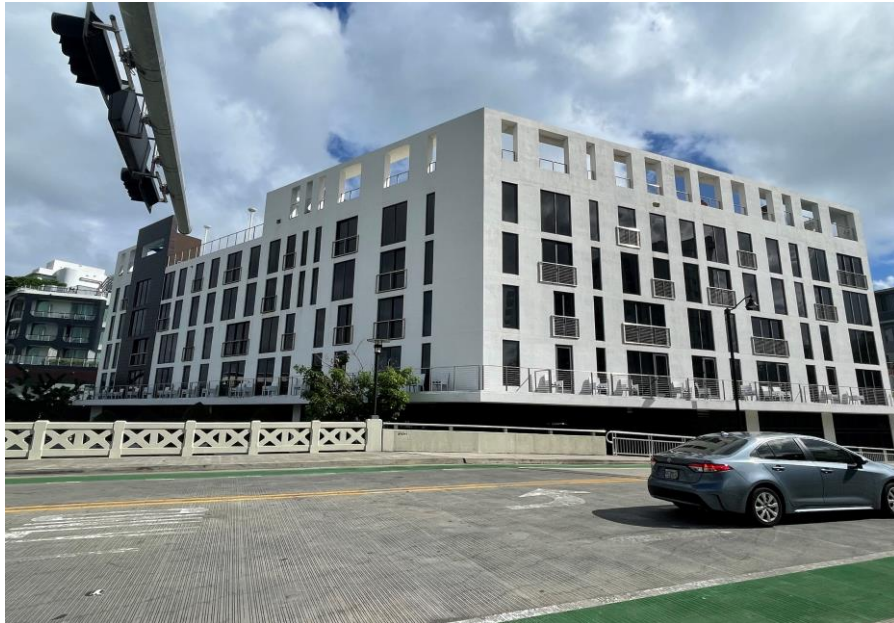
12 WEST AVENUE BRIDGE / ADJACENT HOTEL
