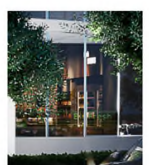
2 ALUMINUM-FRAMED STOREFRONT SYSTEM, W/ IMPACT-RESISTANT GLASS
