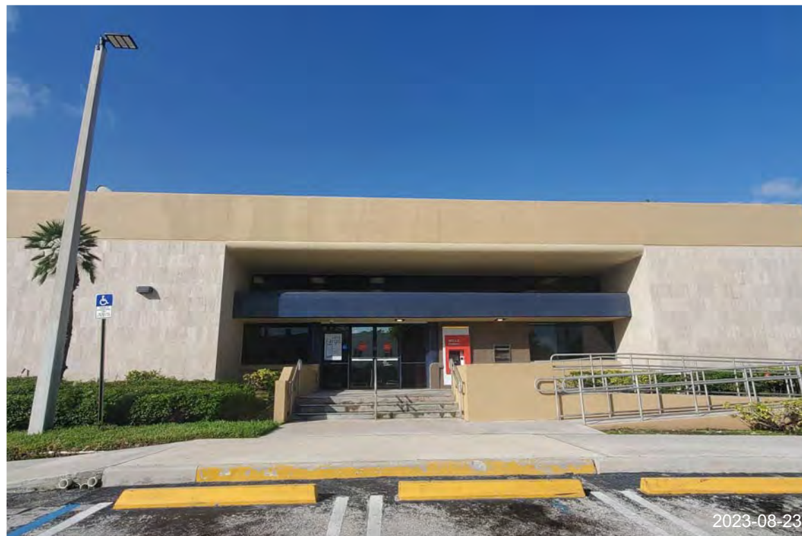
25. VIEW OF WELLS FARGO ENTRANCE FROM EXISTING PARKING
