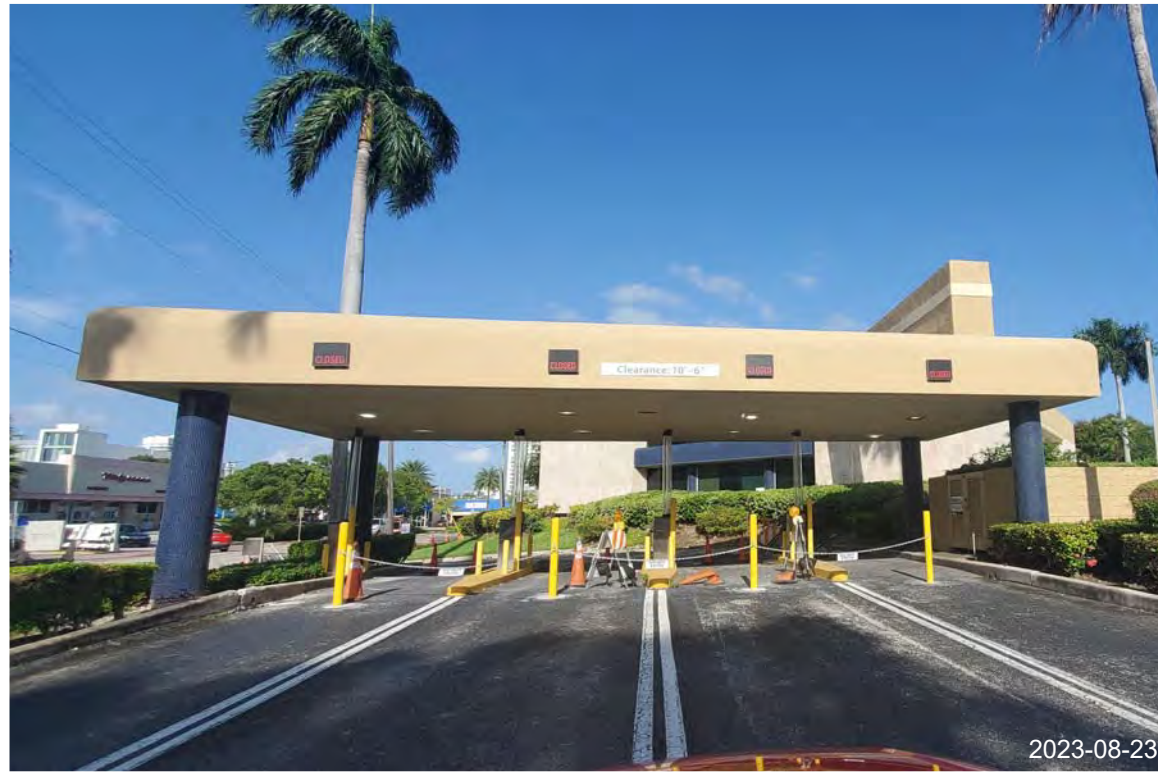
23. EXISTING DRIVE THRU BANK ON SITE
