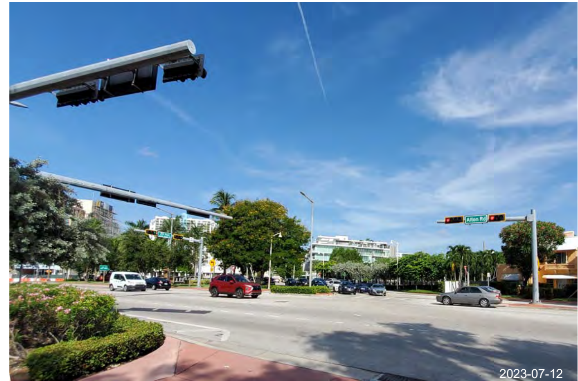
1. VIEW OF ALTON RD FROM NORTH OF SITE
