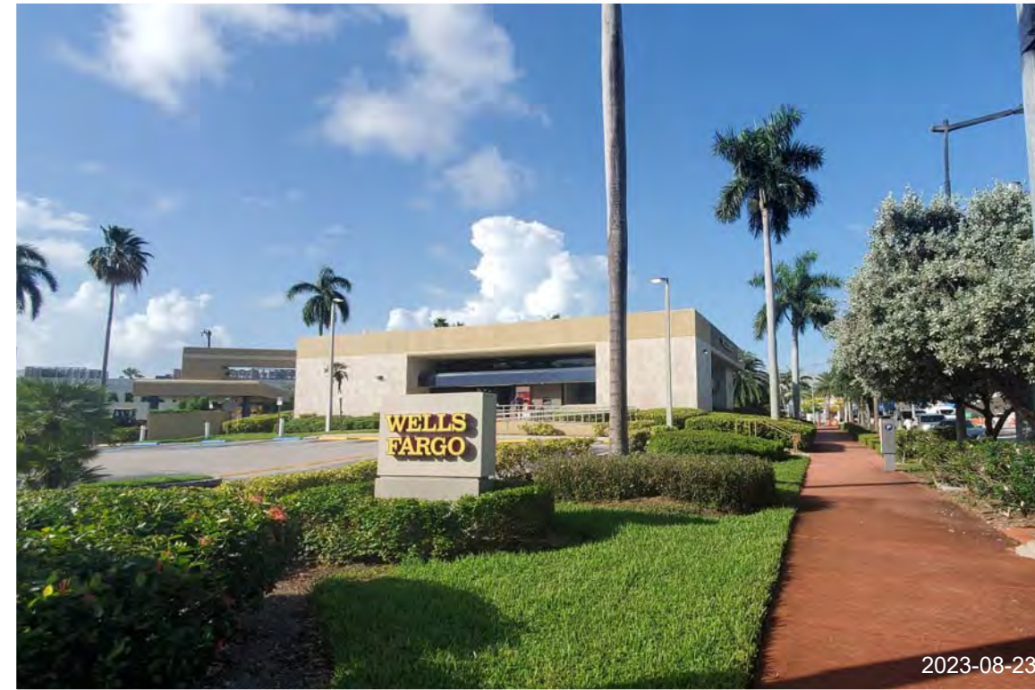
16. EXISTING SITE VIEW FROM SIDEWALK ON ALTON RD.
