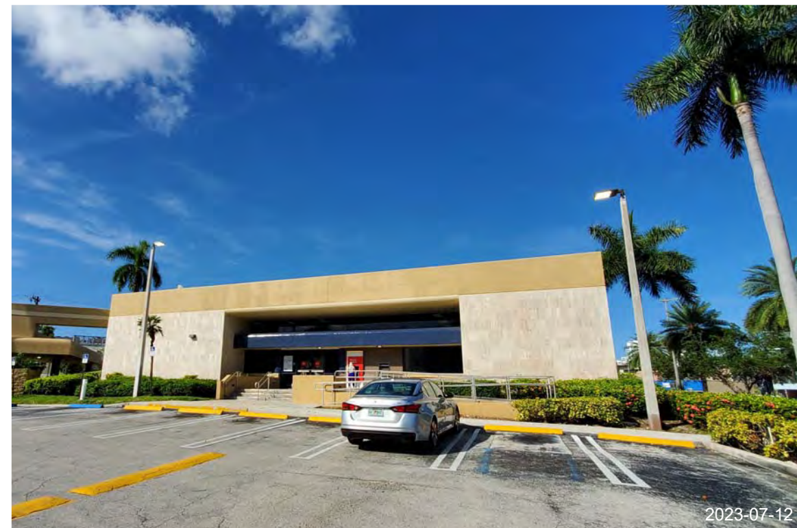
6. VIEW OF EXISTING WELLS FARGO BANK FROM PARKING
