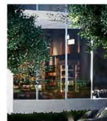
2 ALUMINUM-FRAMED STOREFRONT SYSTEM, W/ IMPCT-RESISTANT GLASS
