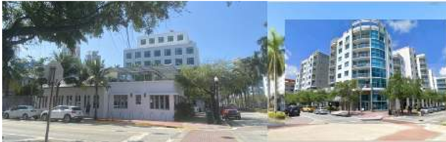
G. CONTEXT PHOTO WASHINGTON AVENUE
