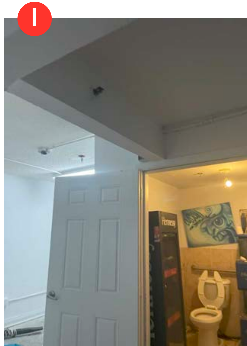
VIEW AT RESTROOM FOR PROPOSED DEMOLITION
