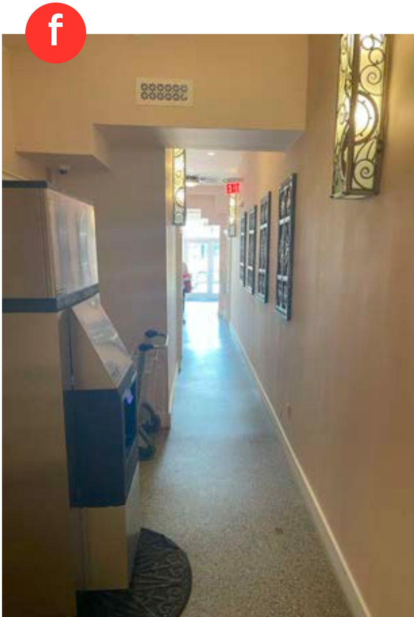
VIEW DOWN CORRIDOR BETWEEN TENANT SEPERATION WALL (RIGHT) AND LOBBY, FACING WEST TOWARDS HOTEL ENTRANCE
