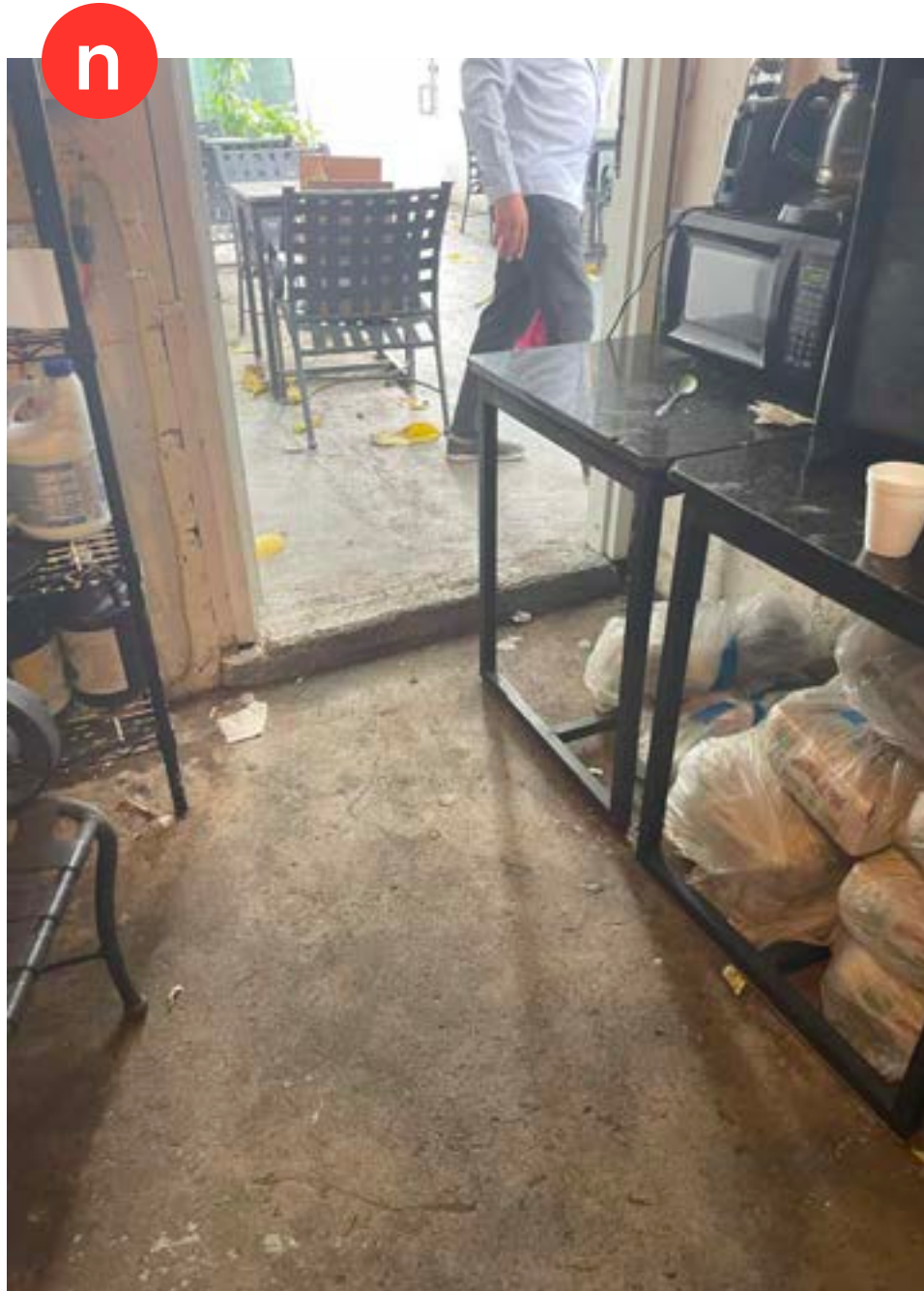
VIEW INSIDE REAR STORAGE ROOM (PROPOSED OUTDOOR COVERED BAR LOCATION)
