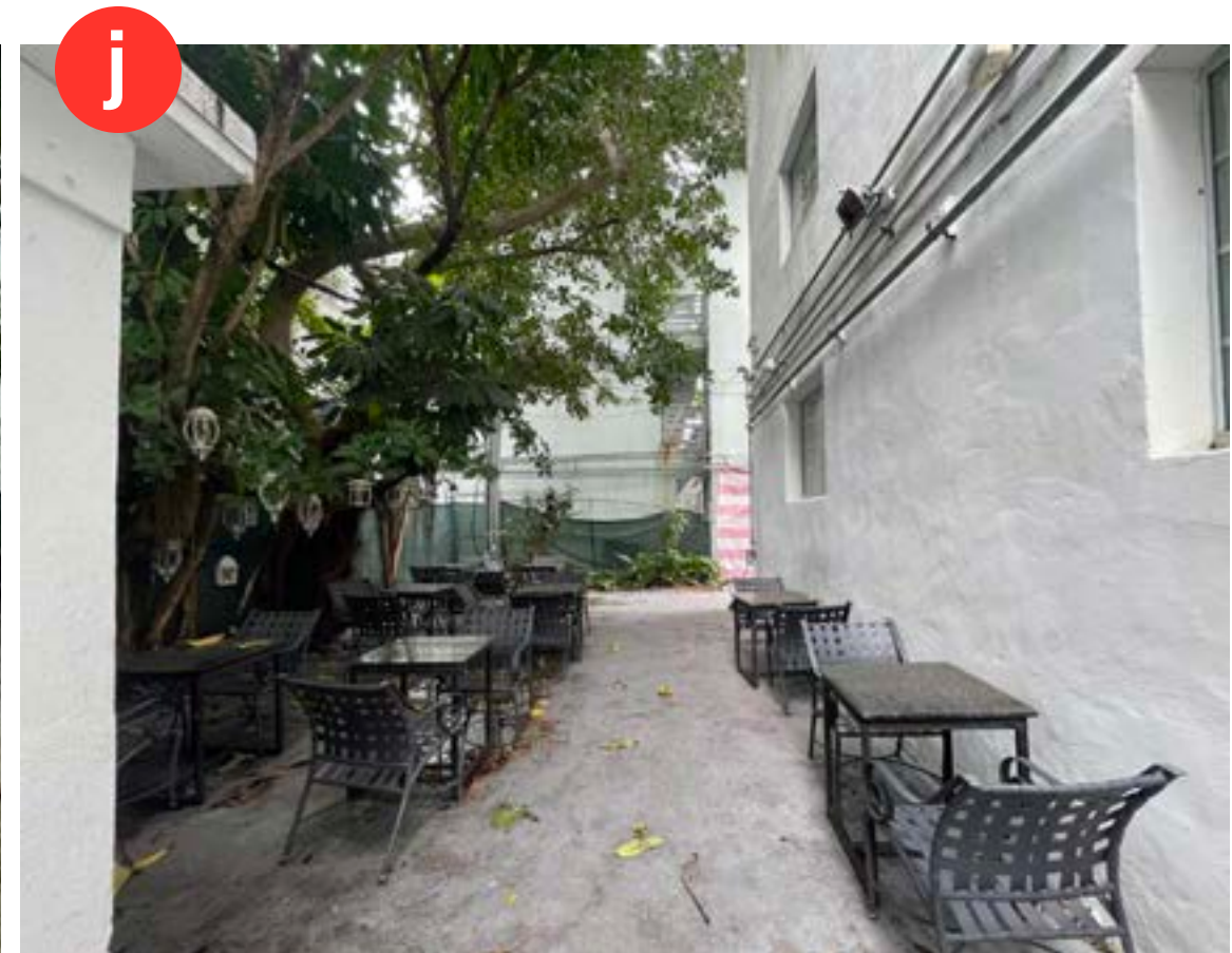
COURTYARD EAST VIEW - STORAGE ROOM ON LEFT
