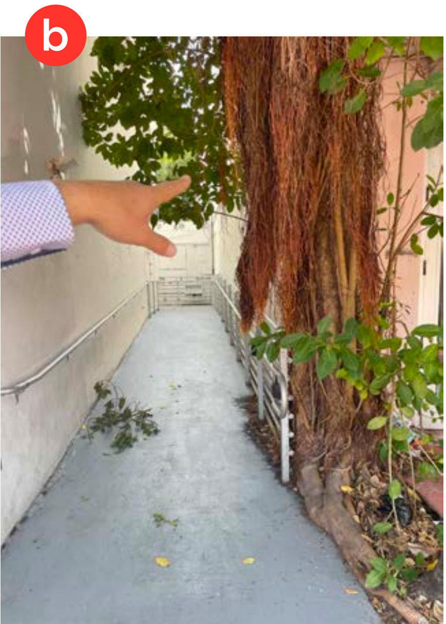
ADJACENT RAMP TO NEIGHBORING Z'OCEAN HOTEL (NORTH SIDE OF PROPERTY)
