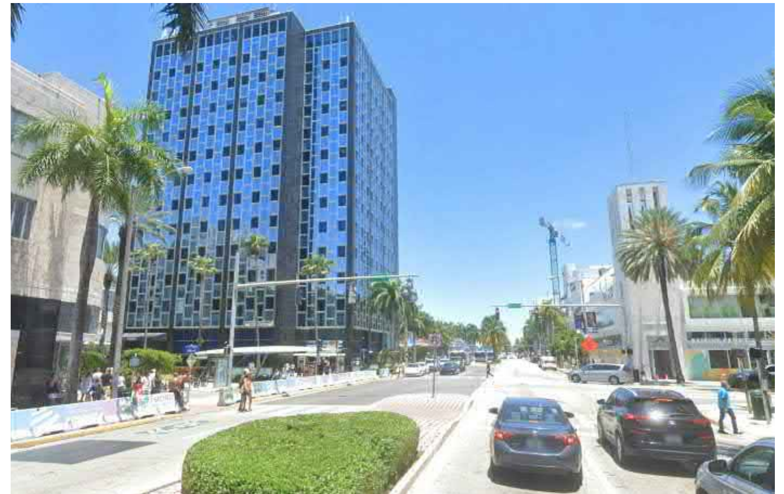
WASHINGTON AVE NORTH VIEW
