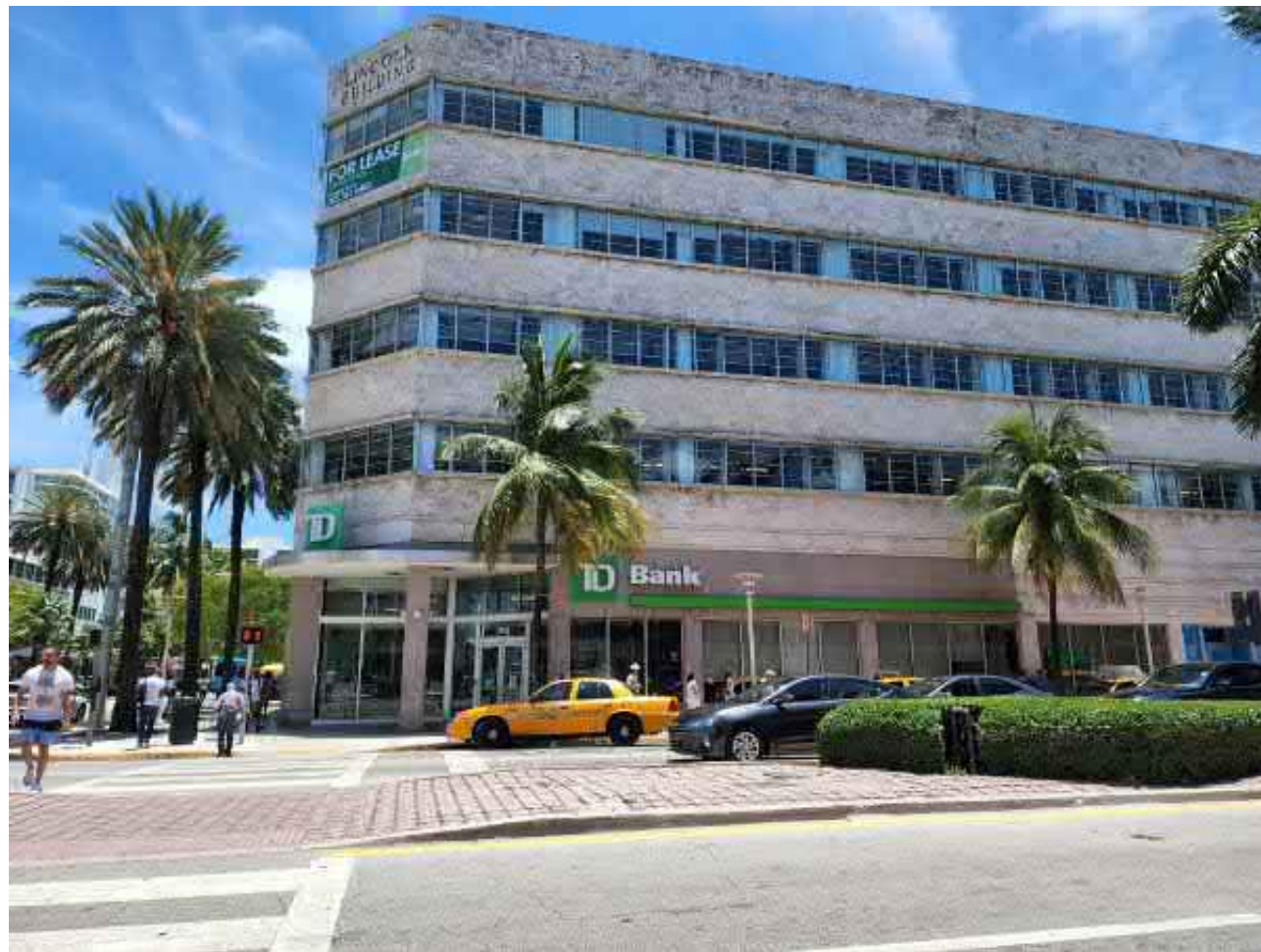
TD BANK OVERALL BUILDING VIEW
