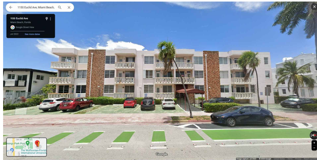
East Elevation OLD RAILINGS(Euclid Ave.)
