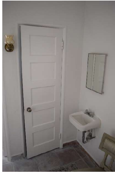
Figure 27. Interior door at Bedroom 2, May 2021.
