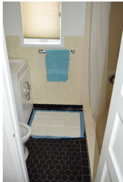
Figure 25. Black hex floor tile and black base at Bath 1, May 2021.
