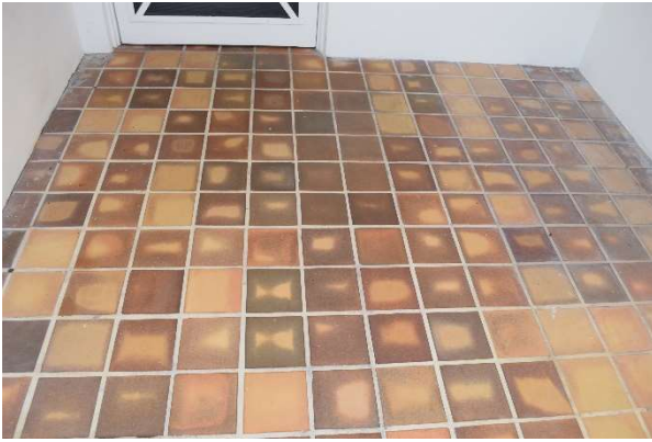
Figure 7. Tile pavers at front porch, May 2021.
