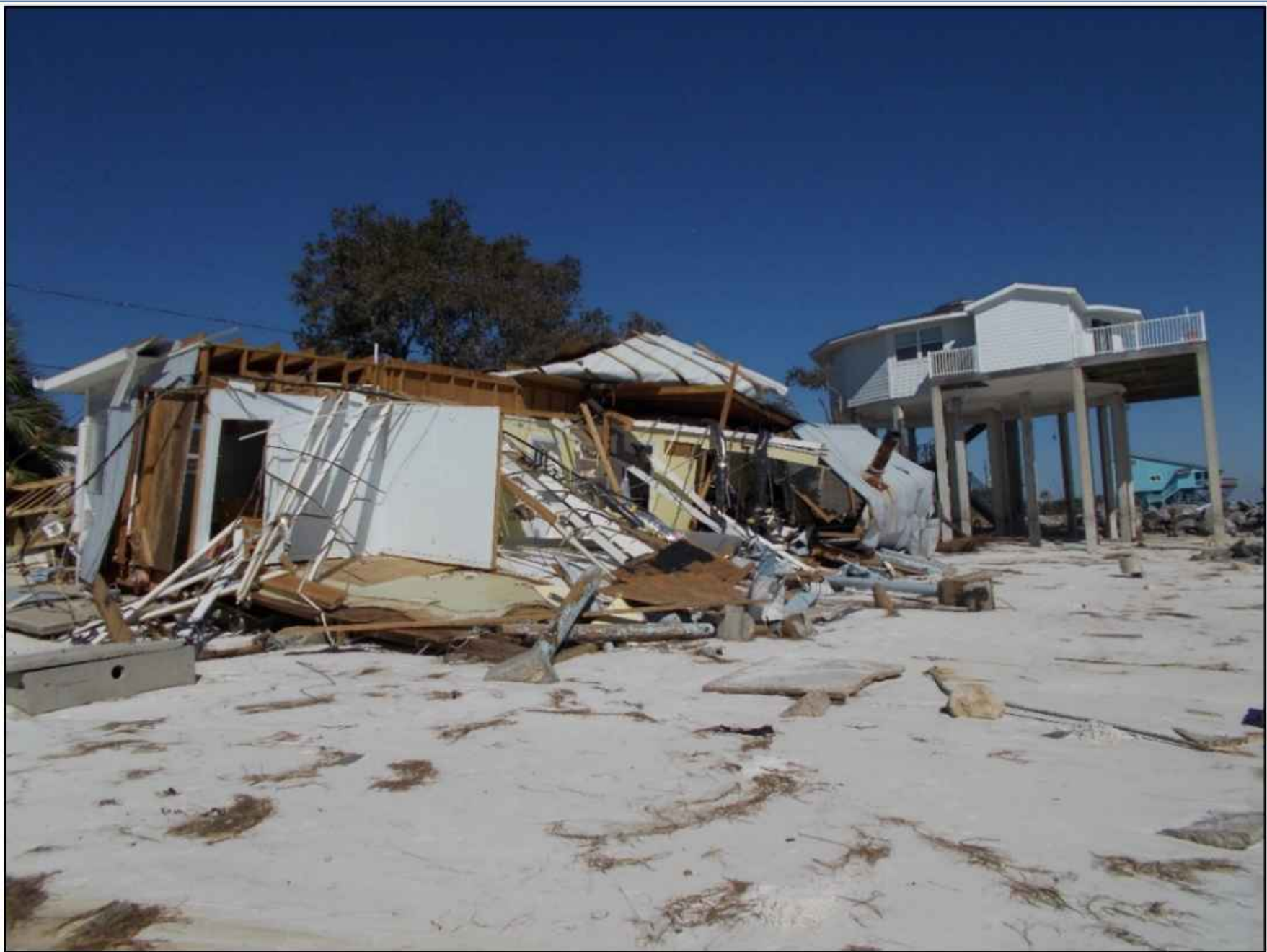
Figure 101. Dwelling destroyed near R211, Southwest Cape.
