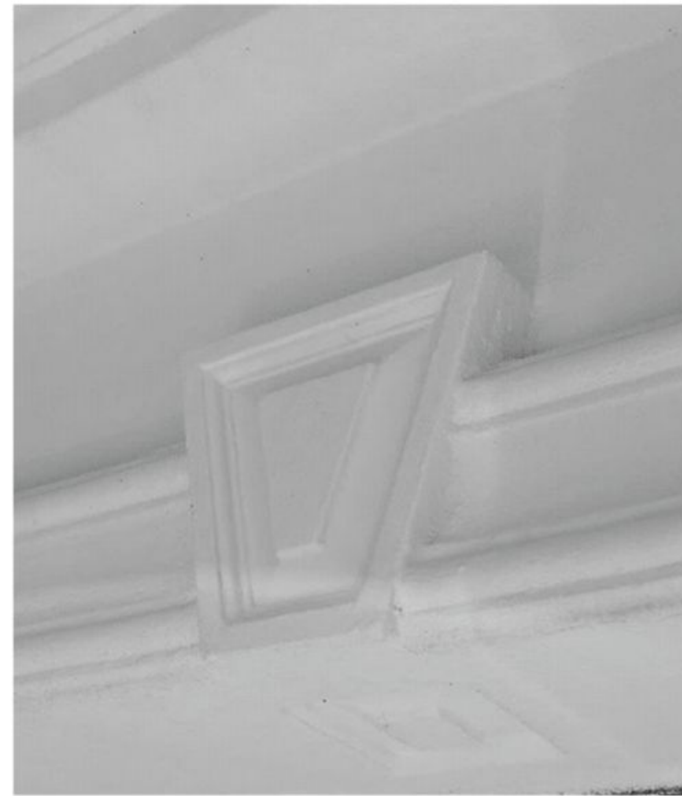
Figure 81. Detail of keystone at garage door, May 2021.
