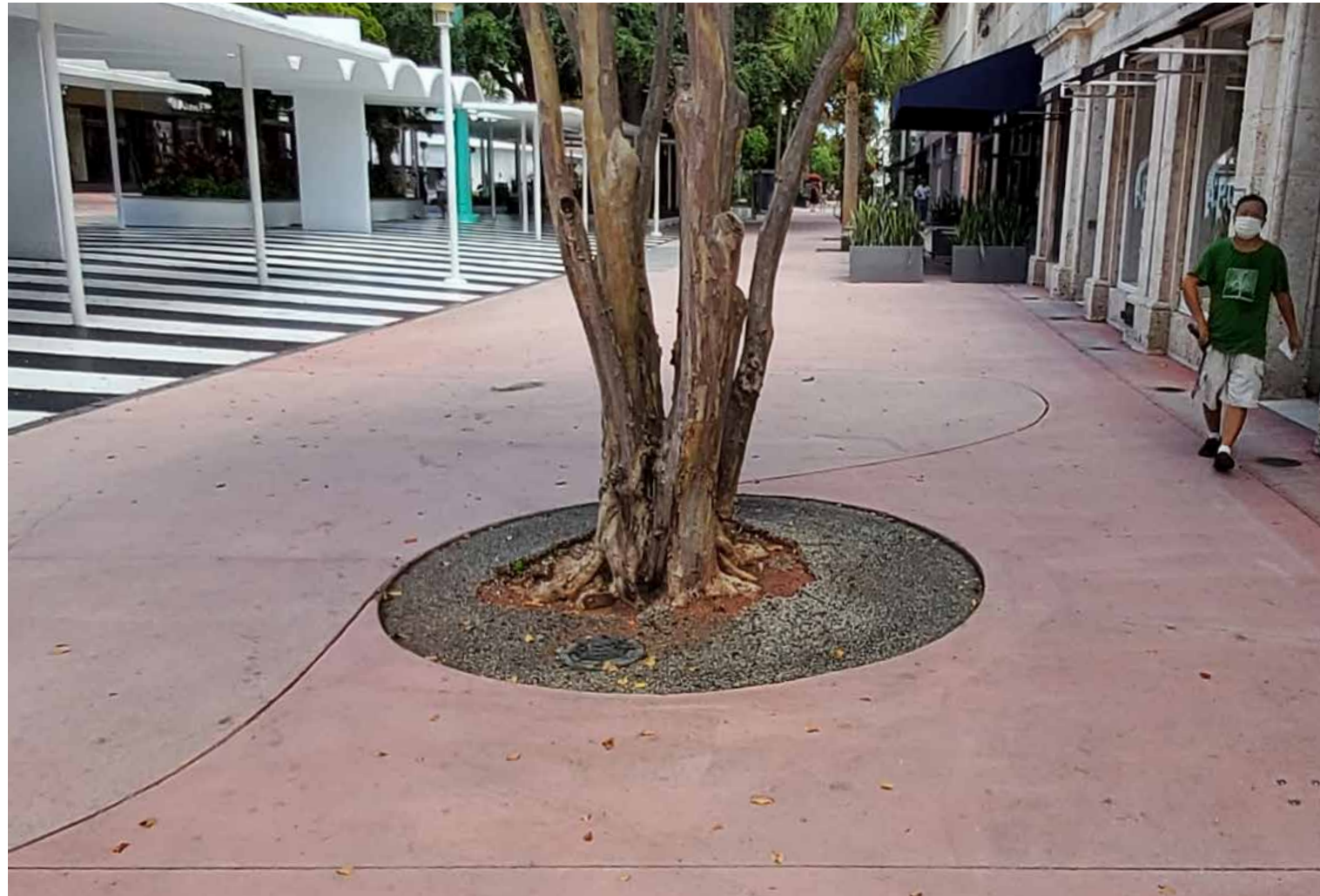
EXISTING PROMENADE TREE PIT AT 1000 BLOCK
