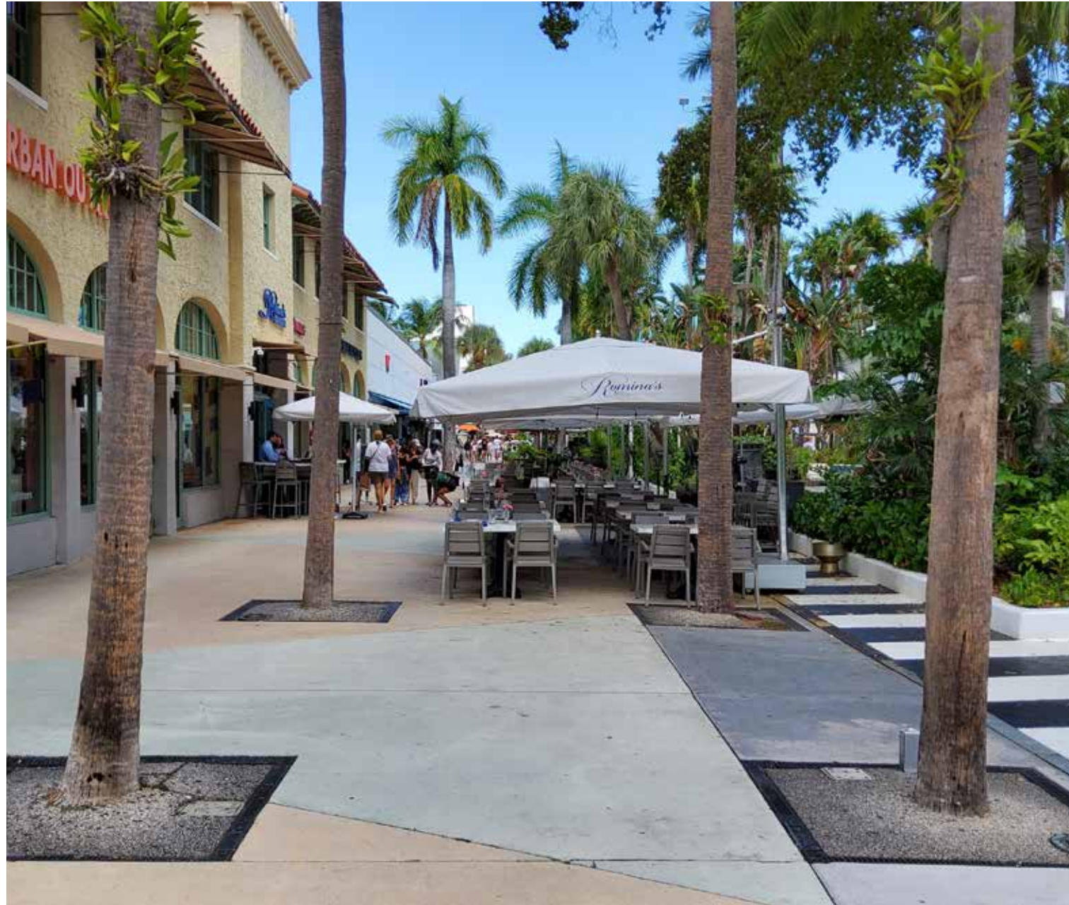
EXISTING TREE PITS WITH WORN RESIN BOND SURFACING AT JEFFERSON AVE. INTERSECTION
