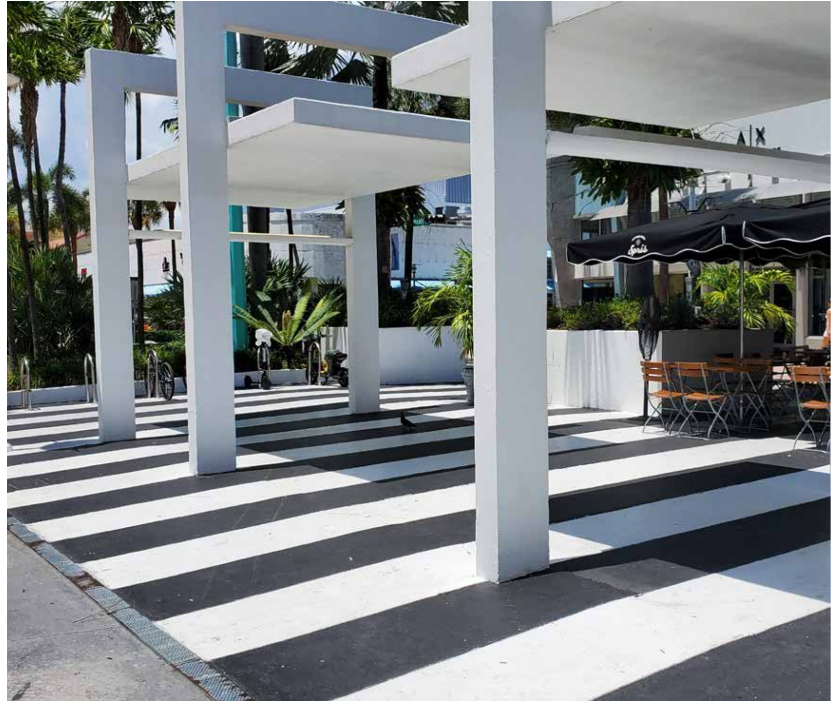
PIANO KEY PAVING AT 700 BLOCK - TODAY
