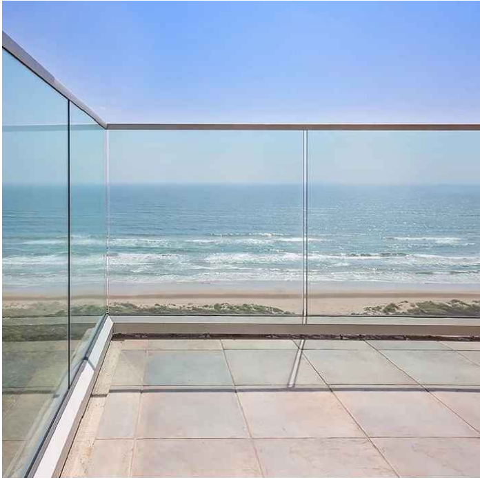
A3 NEW 42" HEIGHT FRAMELESS GLASS GUARDRAIL AT ROOFTOP AND STAIRCASE.
