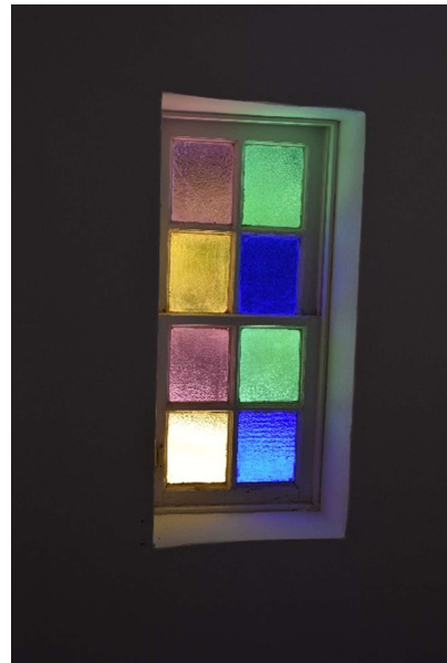
Figure 10. Stained glass window at Stair Hall, May 2021.
