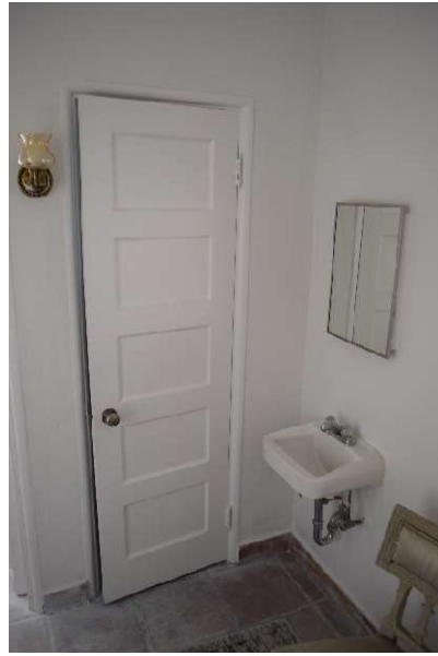
Figure 27. Interior door at Bedroom 2, May 2021.
