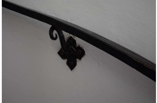
Figure 29. Bracket supporting stair handrail, May 2021.
