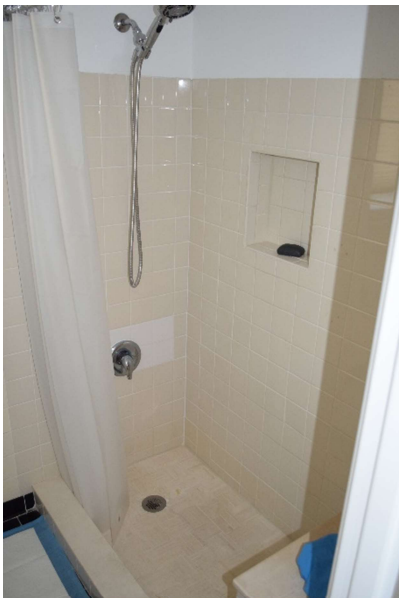
Figure 24. Yellow wall tile at Bath 1, May 2021.
