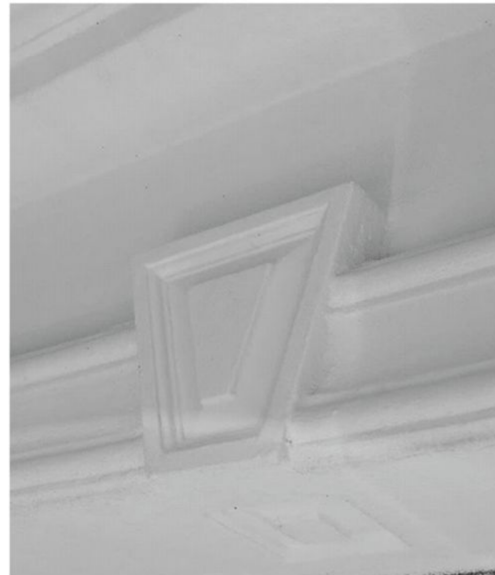
Figure 81. Detail of keystone at garage door, May 2021.
