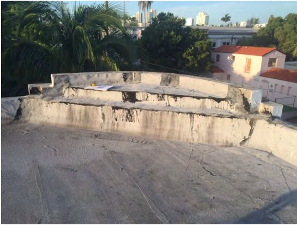
South West Roof pylon support
