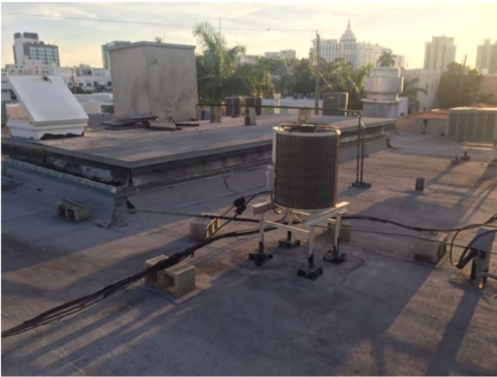
Roof North view
