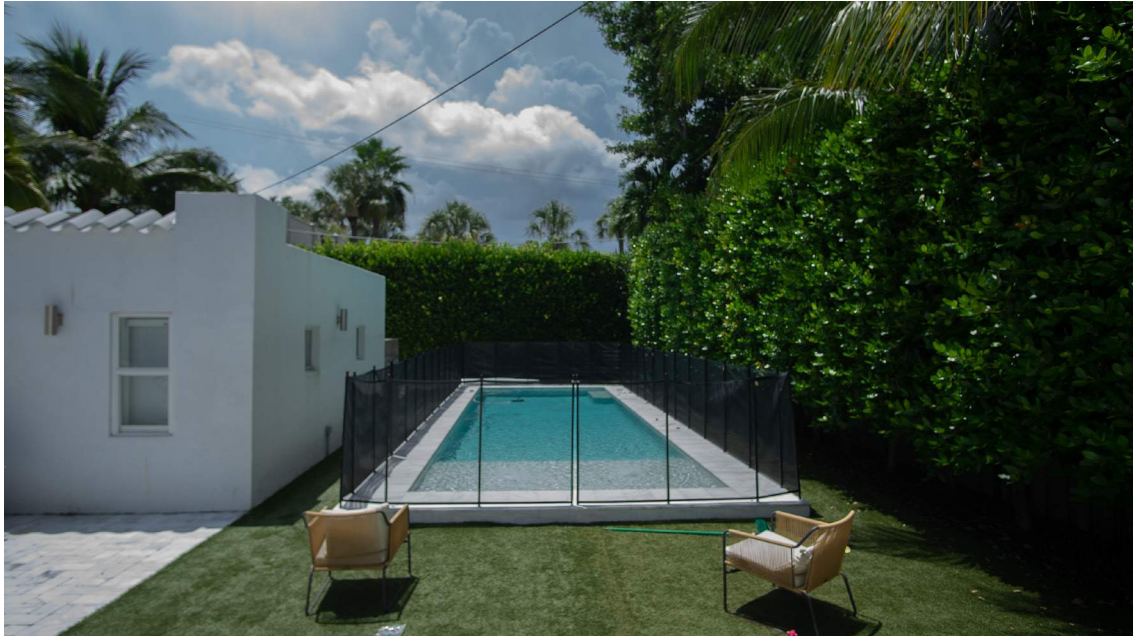
1760 Lenox Ave. Existing rear view of the Pool and Guest House. Picture taken on 8/18/2023
