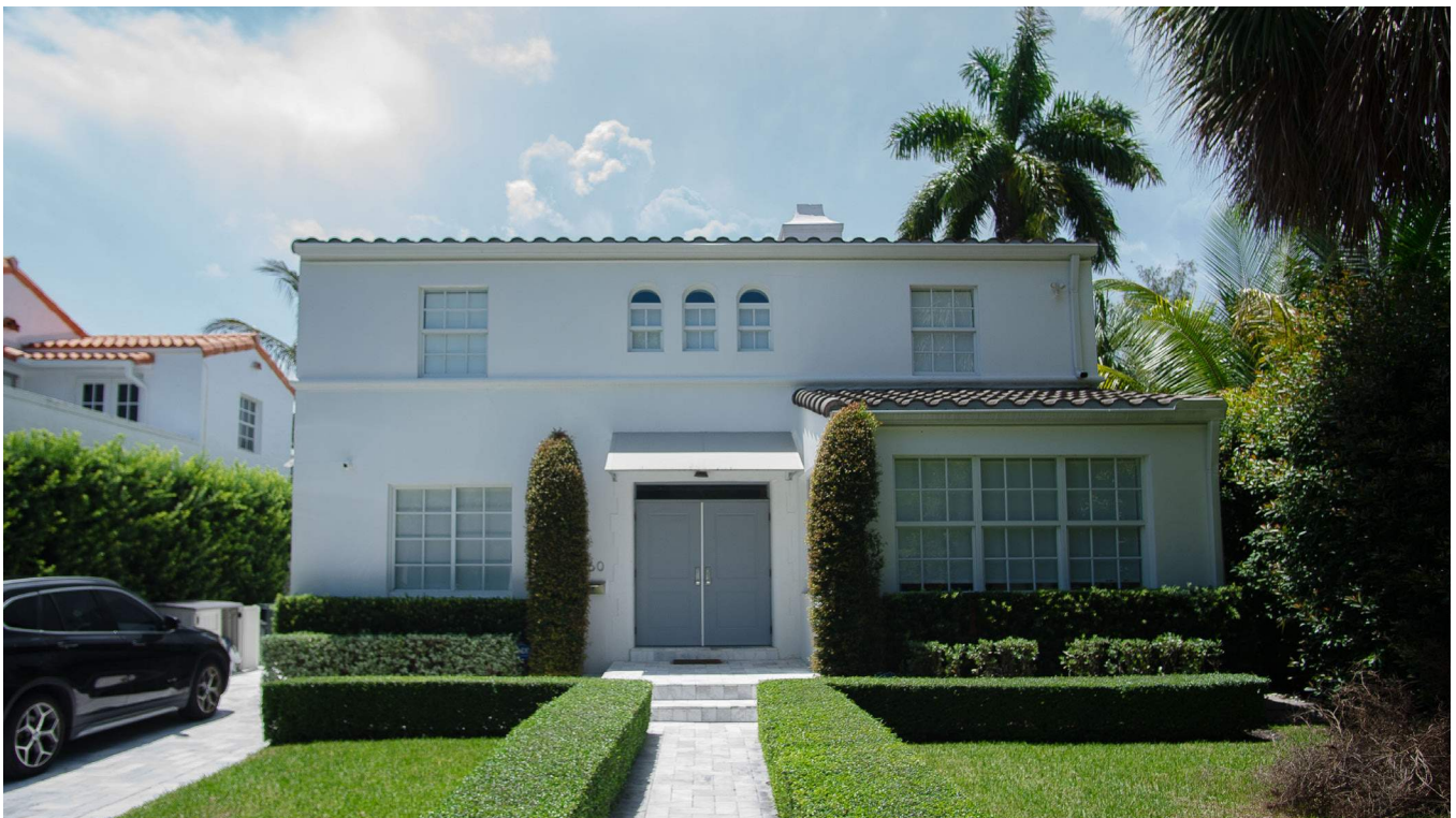
1760 Lenox Ave. Existing Residence Front Photo of Residence. Picture Taken 8/18/2023.
