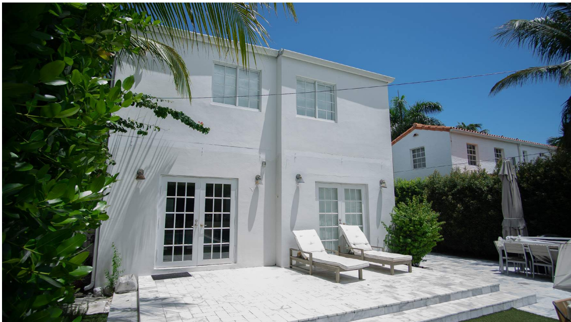
1760 Lenox Ave. Existing rear view of the Residence. Picture taken on 8/18/2023
