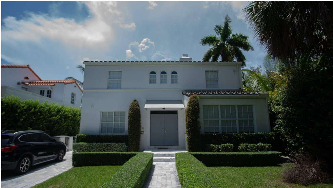
1760 Lenox Ave. Existing front view of the Residence. Picture taken on 8/18/2023
