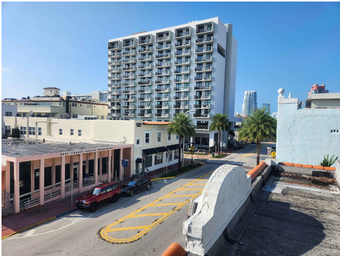
C1 VIEW FROM THE BUILDING ROOFTOP TOWARDS THE INTERSECTION OF COLLINS AVE. AND 6TH STREET PHOTO TAKEN: 06-20-2023
