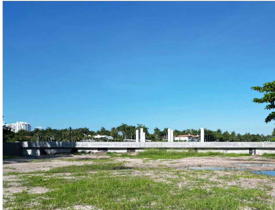
Photograph of existing seawall on site, constructed at T.O.W. height of 8' NGVD
