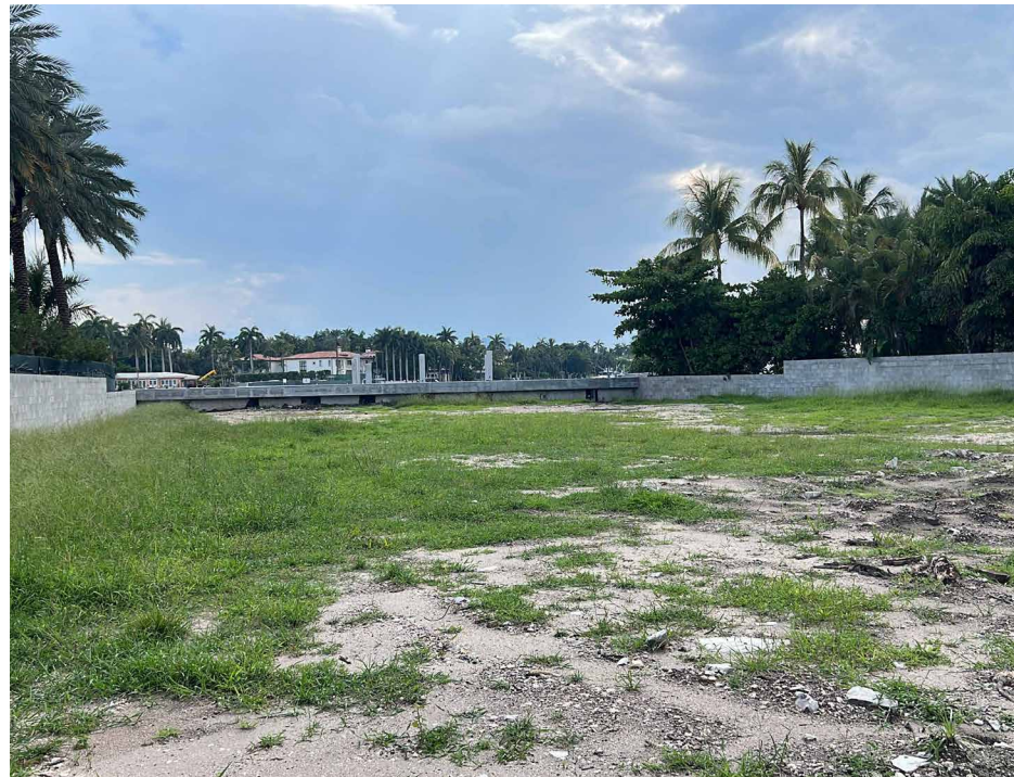
Photograph of existing CMU site walls along north and south boundaries
