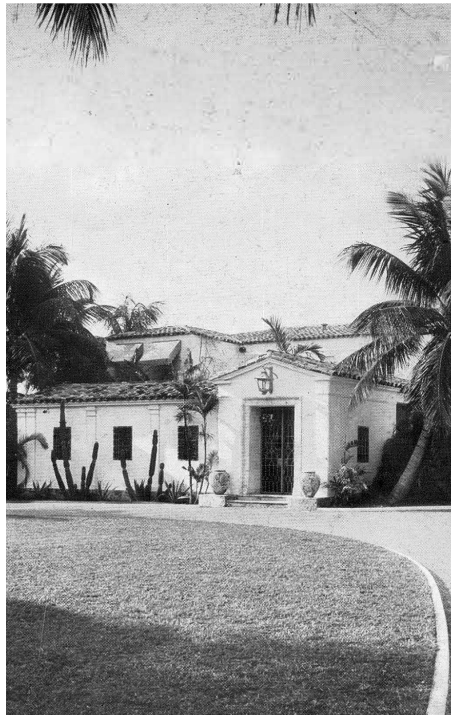
(Image Sourced from (1938). Residence of Mr. George A. Steiner, Sunset Islands, Miami Beach, Florida. Florida Architecture and Allied Arts)
