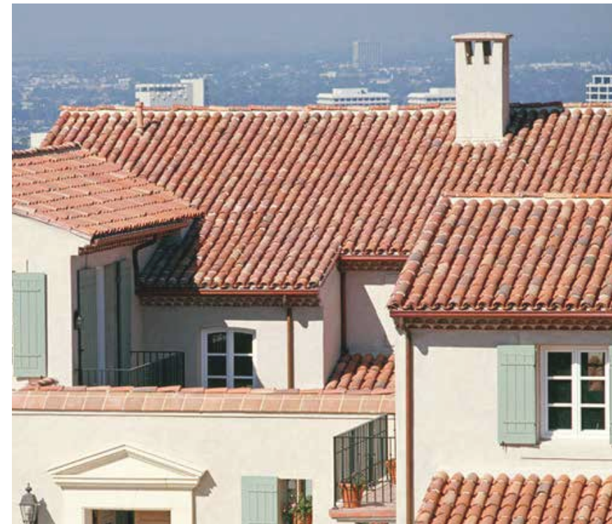
Clay tile roof & Decorative medallion
