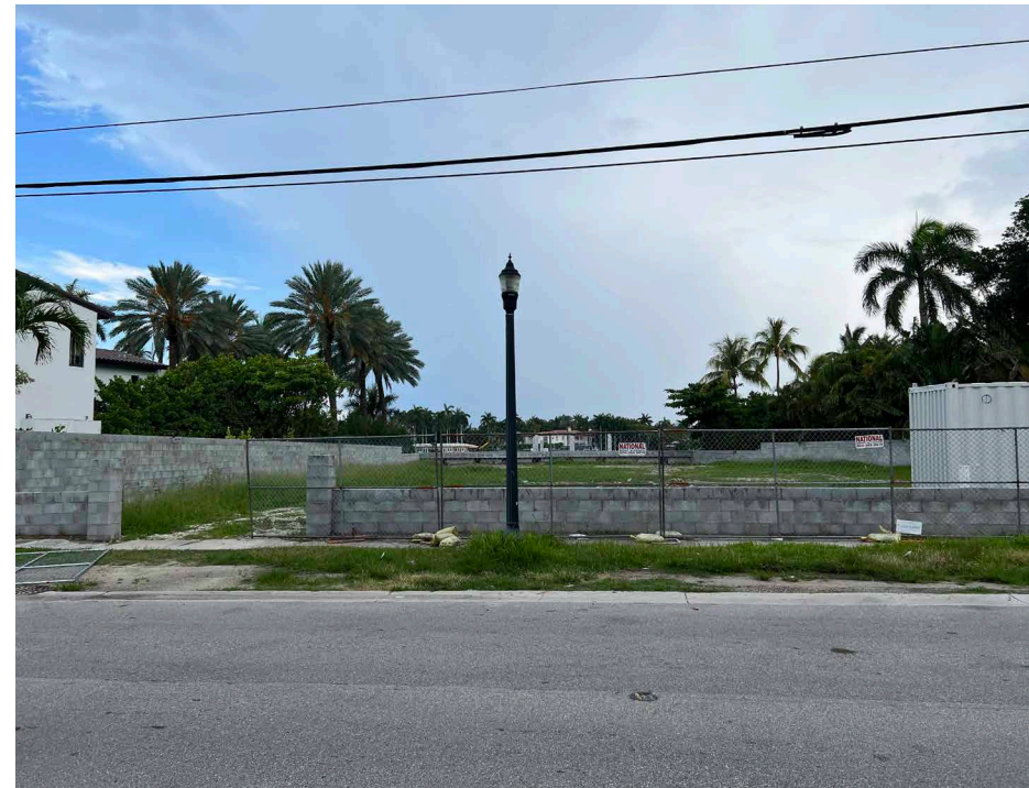
Photograph of existing CMU site wall along eastern site boundary
