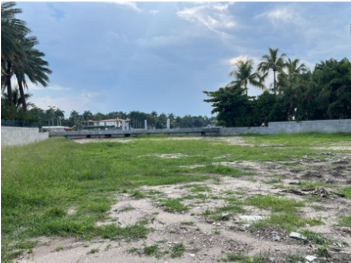
Photograph of existing CMU site walls along north and south boundaries
