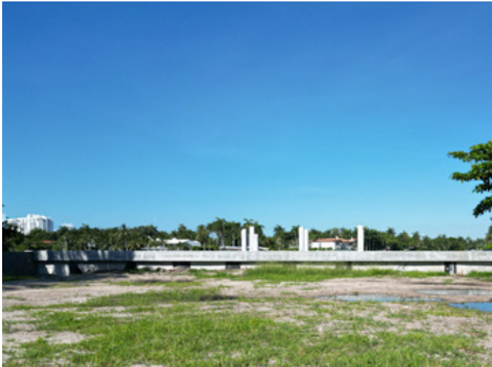
Photograph of existing seawall on the site which is constructed at a T.O.W. height of 8' NGVD
