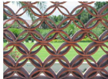
Clay tile brise-soleil.
