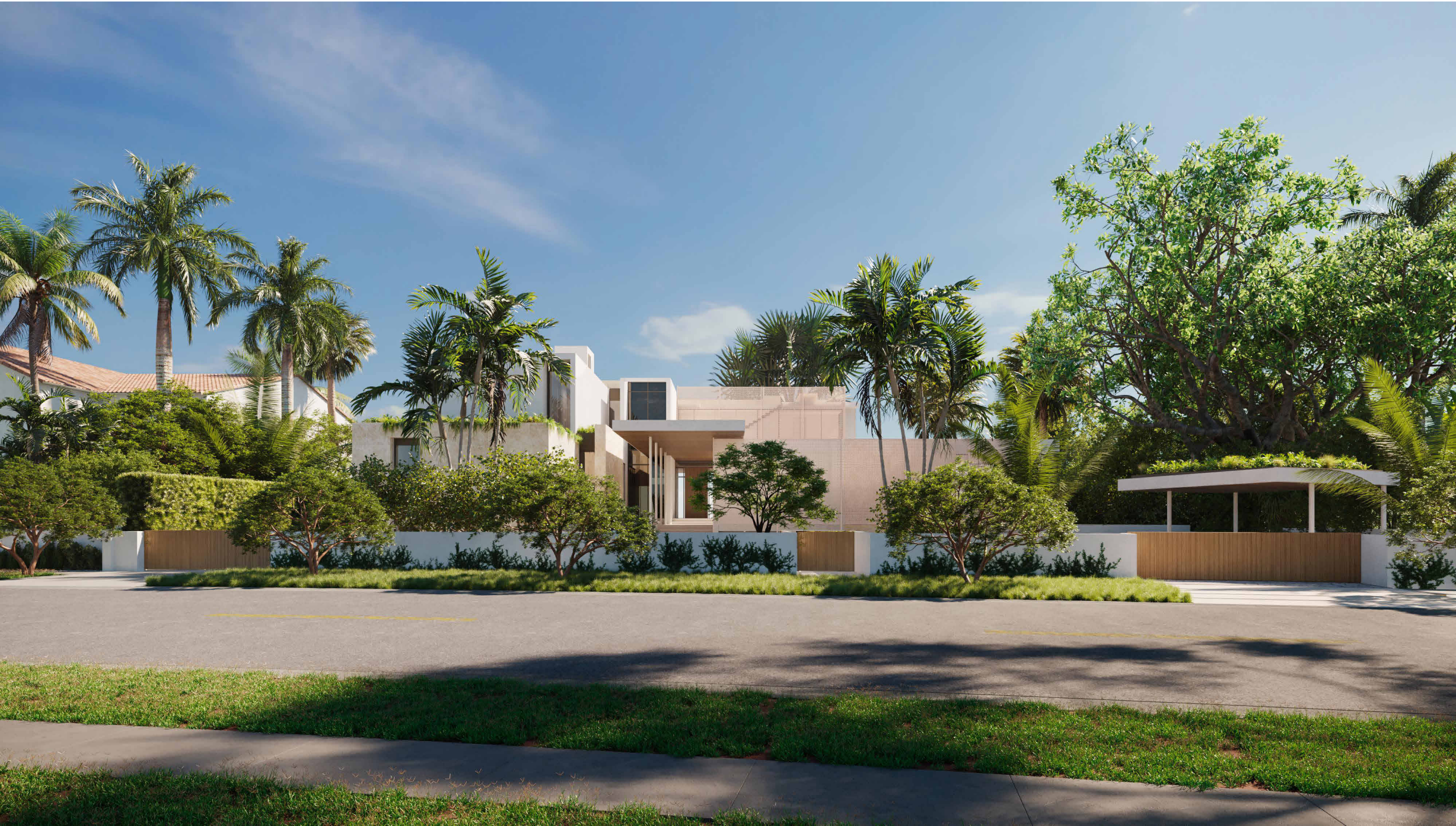
VIEW FROM ACROSS NORTH BAY ROAD
