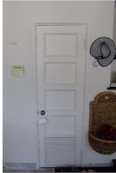
Figure 16. Interior door at Living Room, May 2021.
