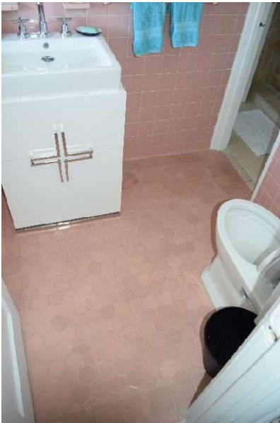
Figure 41. Floor and wall tile at Bath 4, May 2021.
