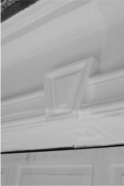
Figure 11. Garage door trim, with keystone, May 2021.
