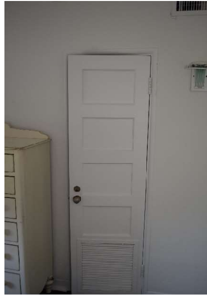
Figure 38. Interior closet door at Bedroom 4, May 2021.
