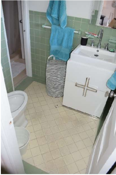
Figure 35. Floor and wall tile at Bath 3, May 2021.
