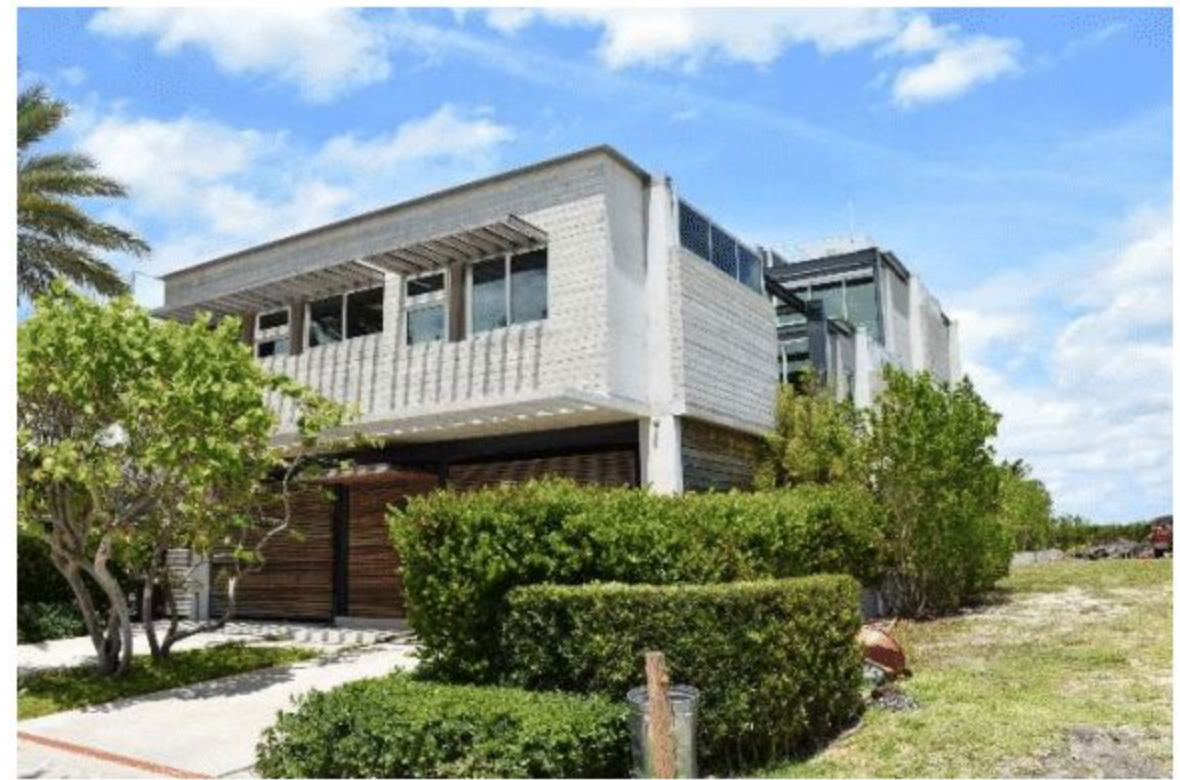
Figure 39. 7709 Atlantic Way (constructed 2019), May 2021.
