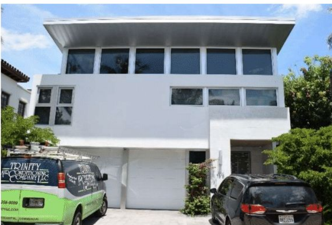
Figure 32. 7815 Atlantic Way (constructed 2015), May 2021.
