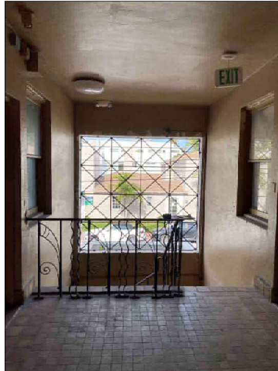
VIEW 2 CORRIDOR WEST VIEW
