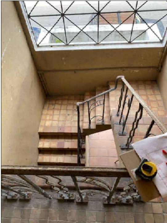
VIEW 4 STAIR WEST VIEW
