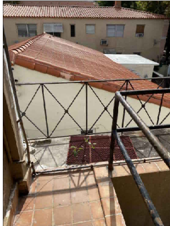
VIEW 5 BALCONY EAST VIEW
