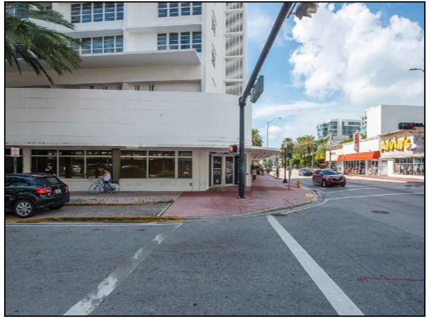
4 VIEW EAST SIDE OF LINCOLN RD
