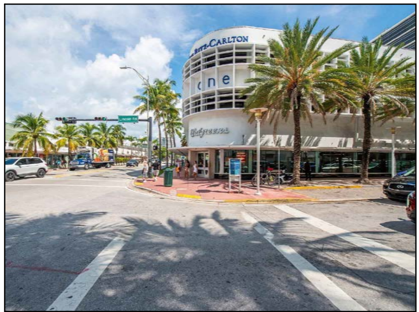
1 VIEW FROM BEACH ACCESS
