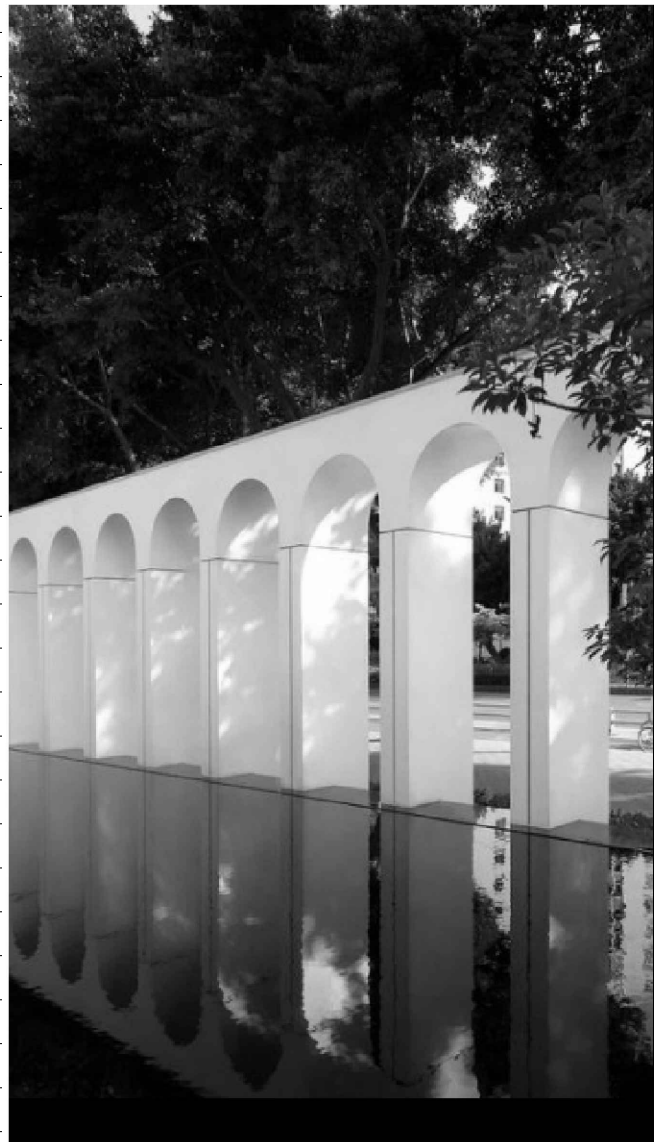
ARCH STRUCTURES + PLANTERS
