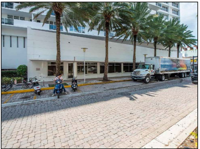
3 BEACH ACCESS WEST SIDE VIEW
