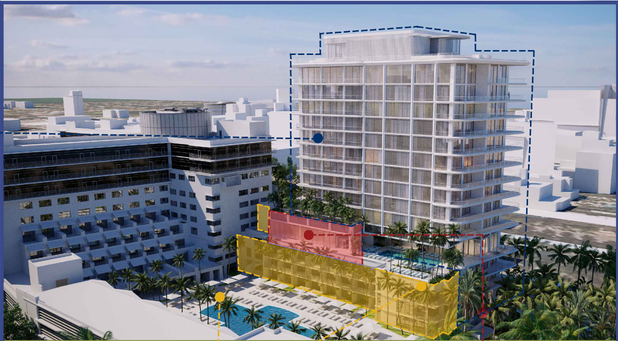
9. New Tower over existing cabana building.
