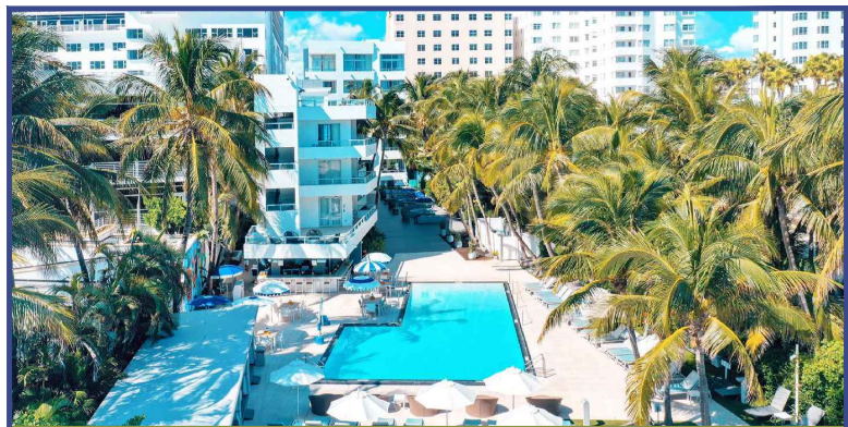
5. Pool Deck (existing)
