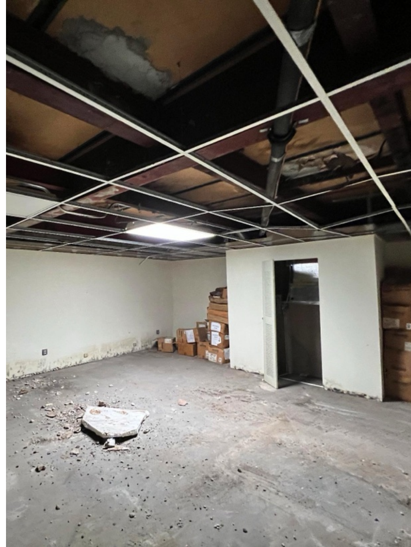
8. Interior at Mezzanine Level
