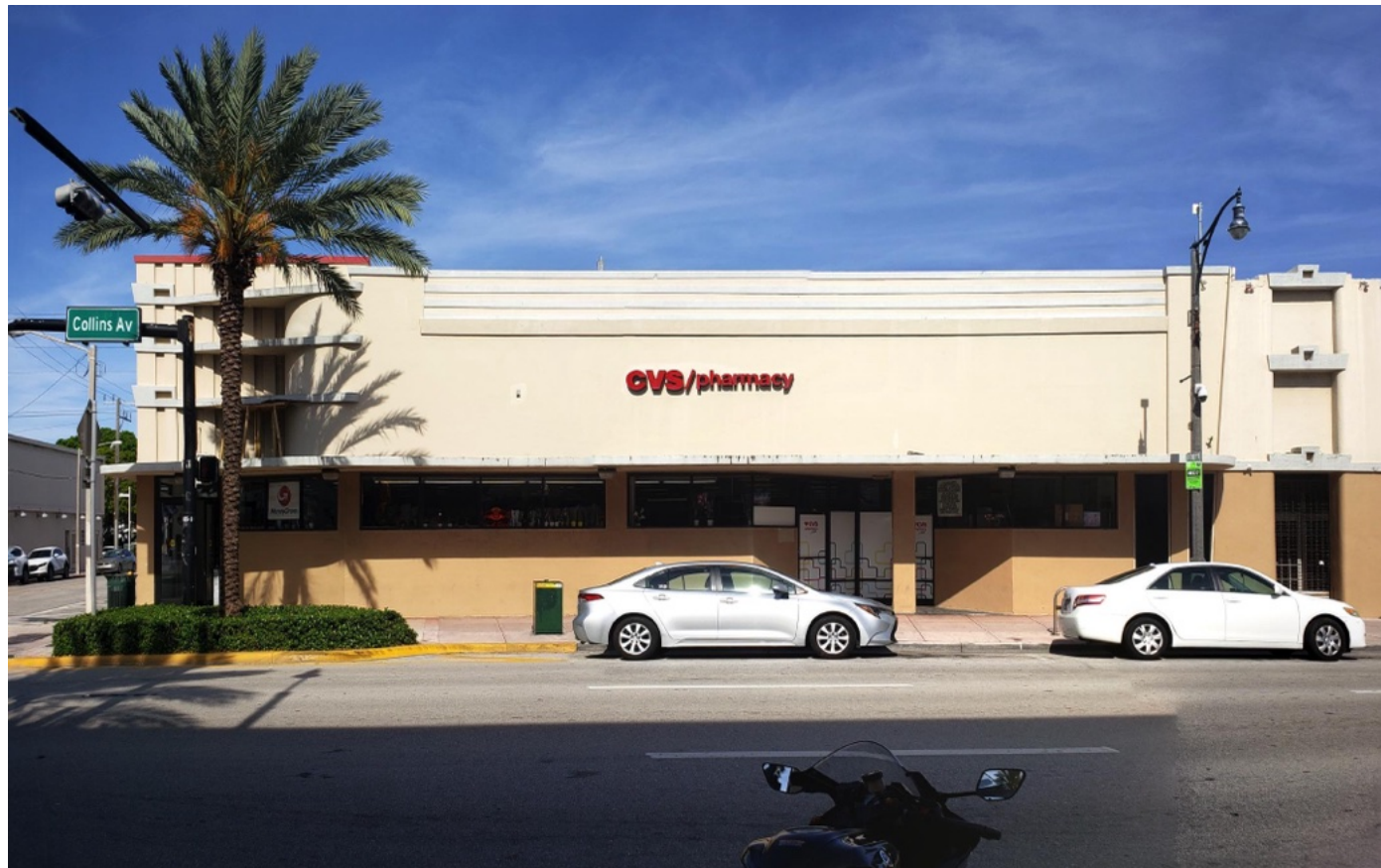
14. COLLINS AVE - EXISTING CVS
