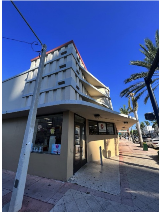
4. STORE ENTRANCE AT CORNER OF COLLINS AVE AND 74TH ST
