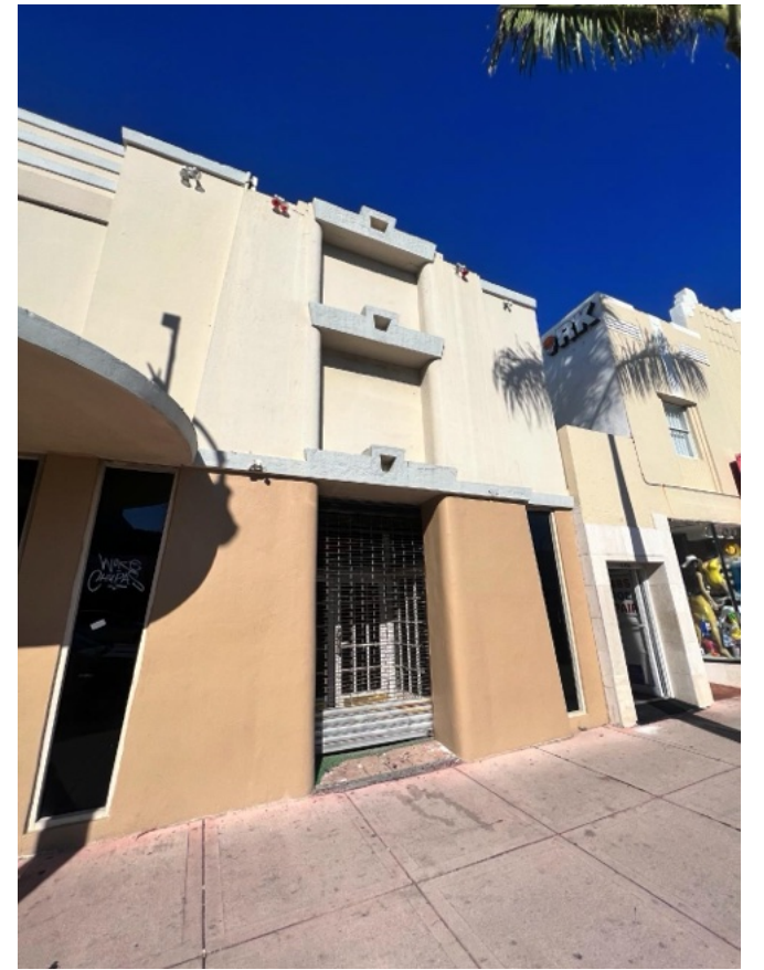
6. CVS - ENTRANCE ON COLLINS AVE
