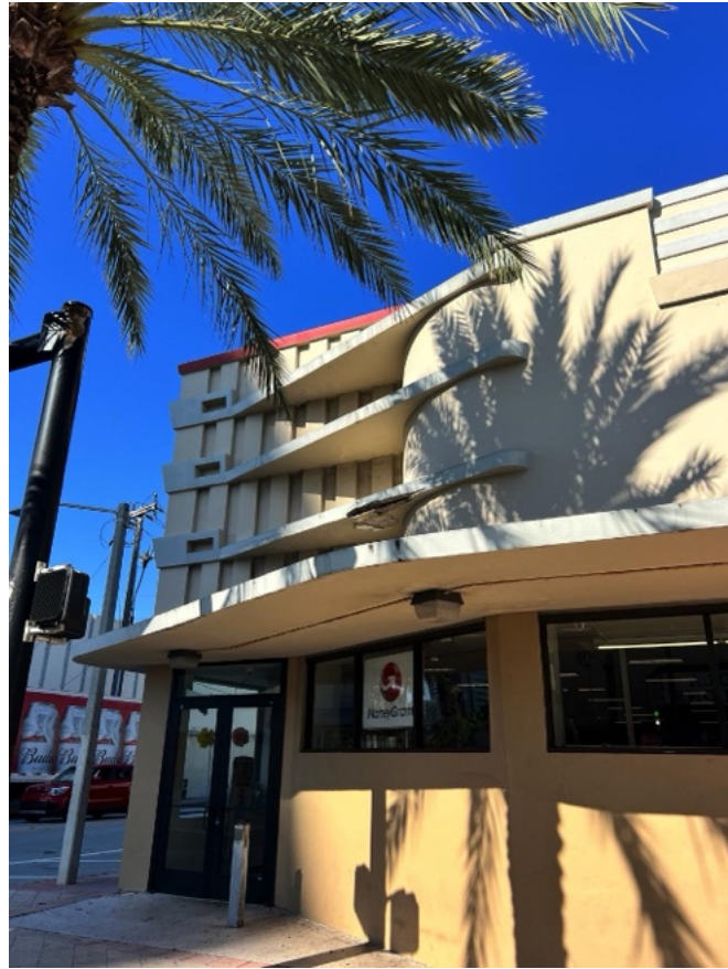
3. CVS - INTERSECTION OF COLLINS AVE AND 74TH ST
