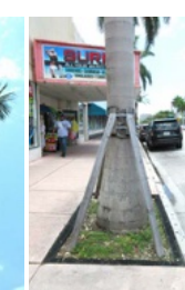
Tree #19 is a Royal Palm street tree located along Collins Avenue. It is growing in a 5ft by 8ft wide sidewalk cut-out. The tree is in fair condition. Braces are on the trunk and the trunk is penciling. Remove the braces before they injure the trunk.
