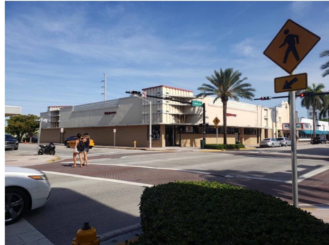
1. CVS - INTERSECTION OF COLLINS AVE AND 74TH ST
