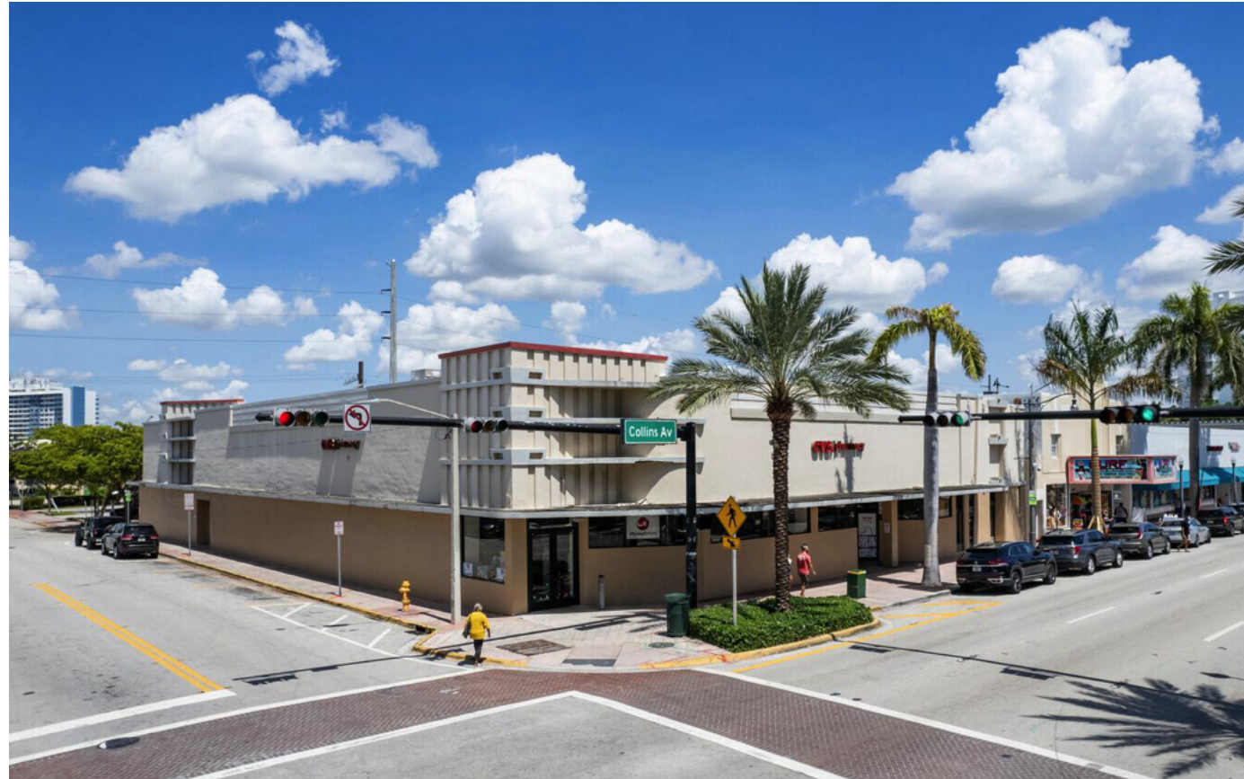
2. CVS - INTERSECTION OF COLLINS AVE AND 74TH ST
