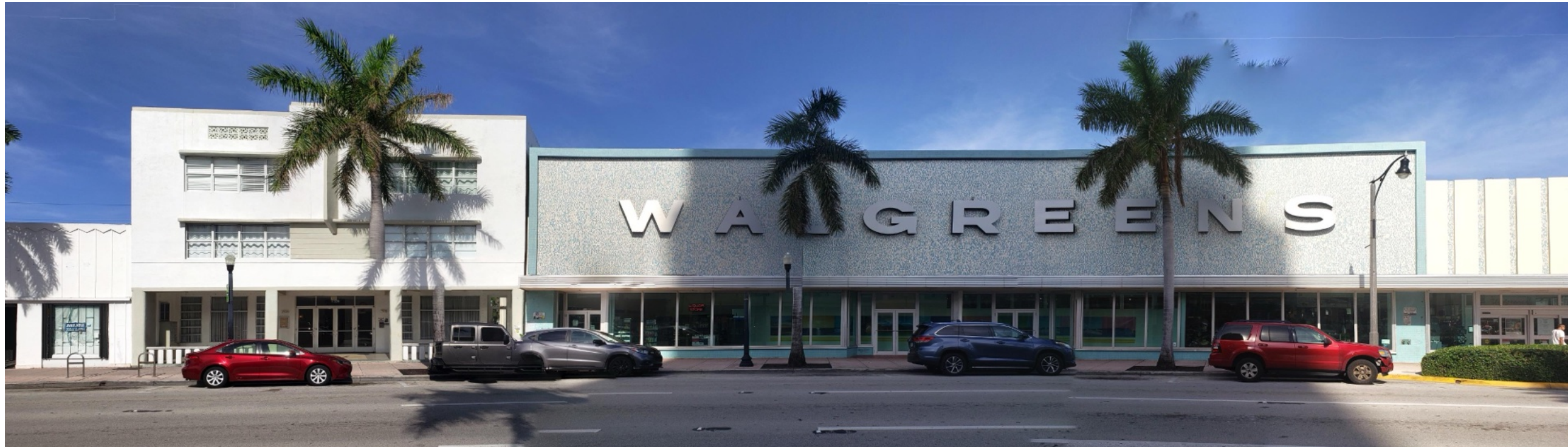
13. COLLINS AVE - ADJACENT WALGREENS
