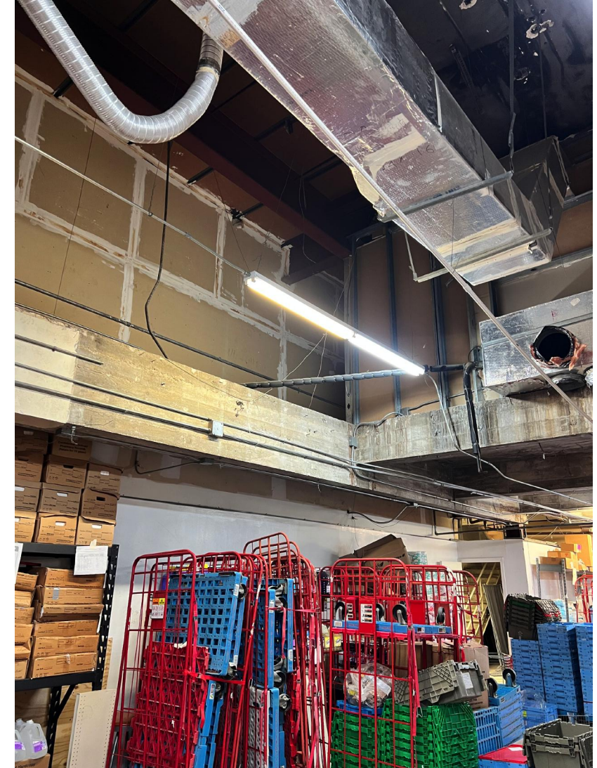
9. Storage Room at Ground Level
