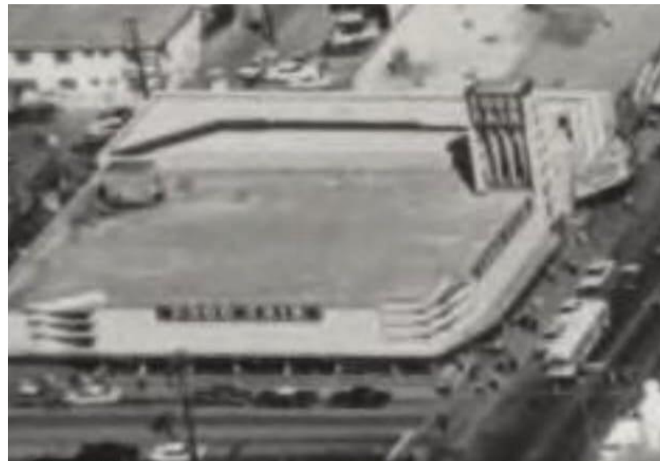
Aerial View of Food Fair Building 1950s
