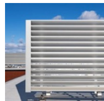
3 MECHANICAL SCREEN WITH METAL LOUVERS
