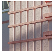
9 HISTORIC RESTORED FLUTED CONCRETE
