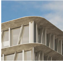
1 CUSTOM POURED CONCRETE SLAB
