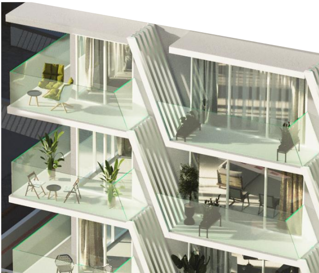
12 SLANTED ALUMINUM BALCONY LOUVERS
