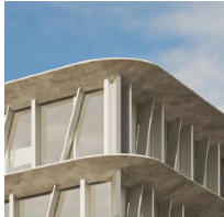
1 CUSTOM POURED CONCRETE SLAB
