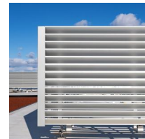
3 MECHANICAL SCREEN WITH METAL LOUVERS
