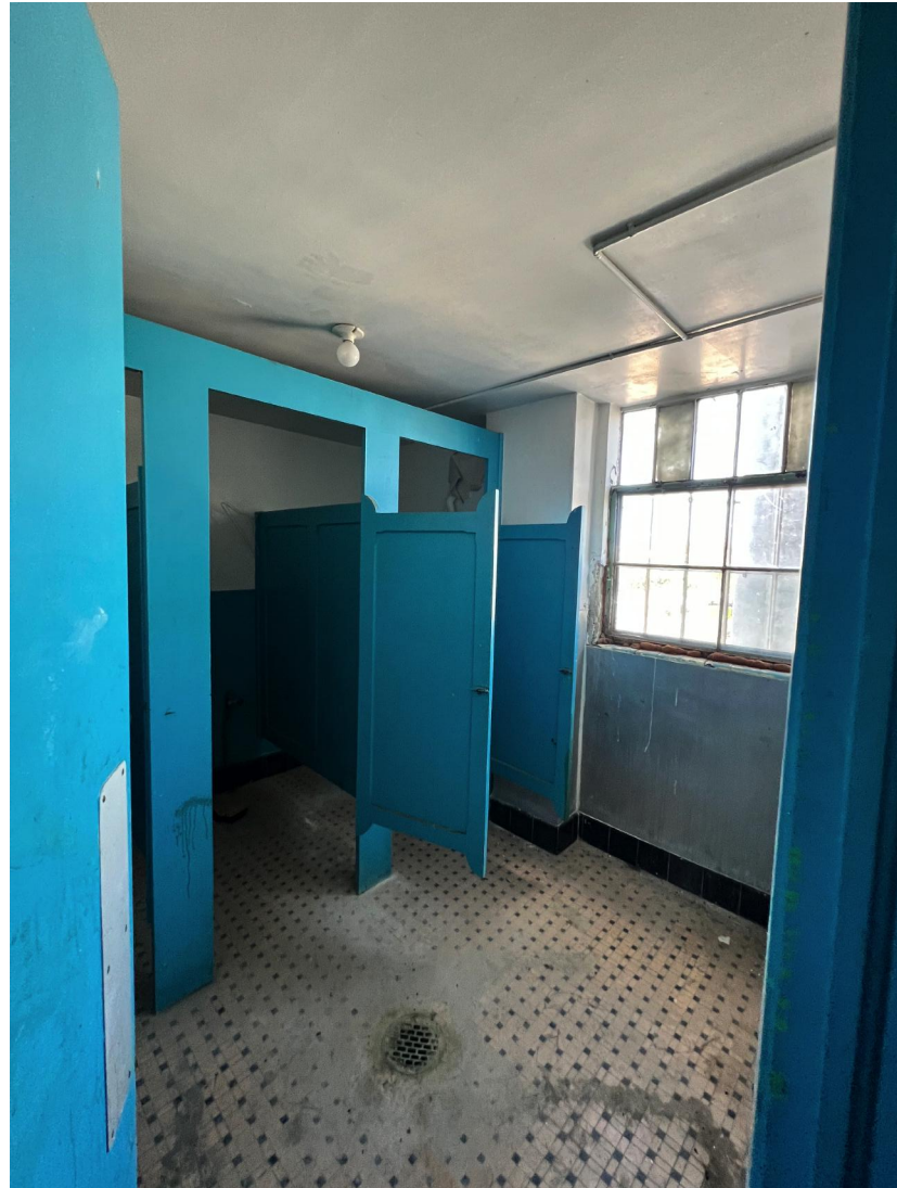
7. Restrooms at Mezzanine Level
