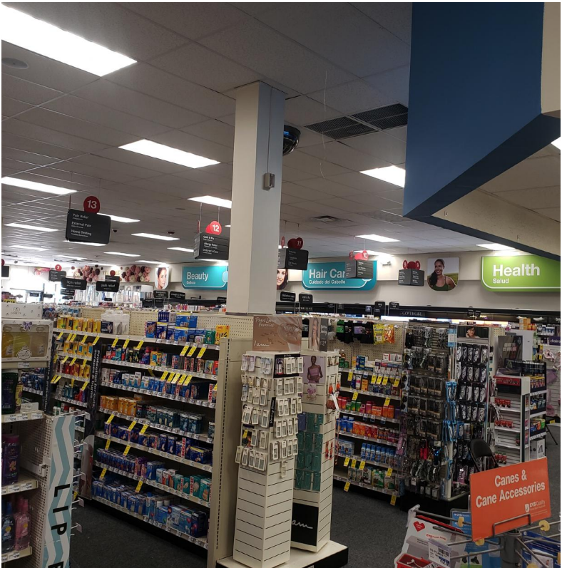
12. CVS Interior- Structural Column
