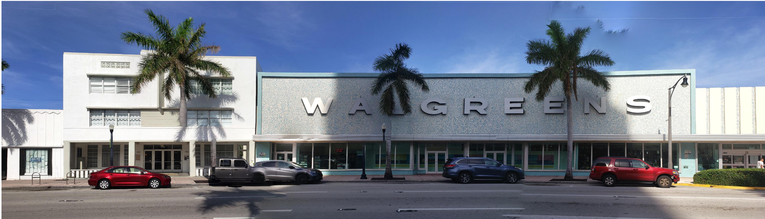
13. COLLINS AVE - ADJACENT WALGREENS
