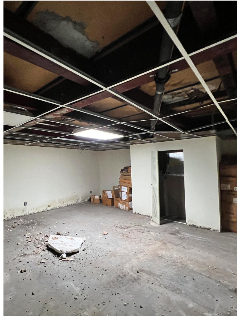
8. Interior at Mezzanine Level
