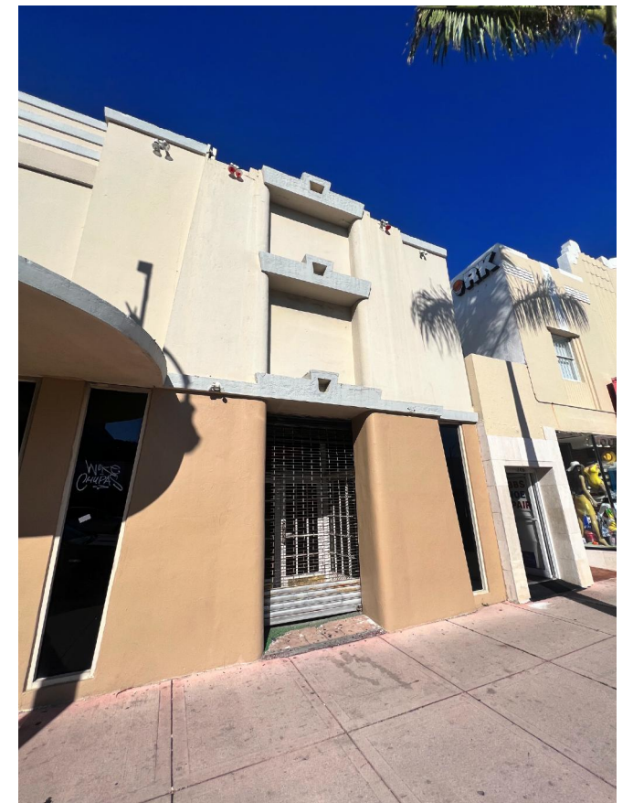
6. CVS - ENTRANCE ON COLLINS AVE
