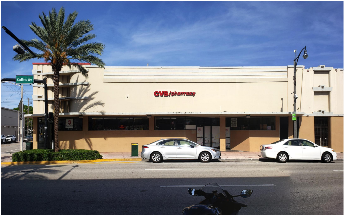
14. COLLINS AVE - EXISTING CVS
