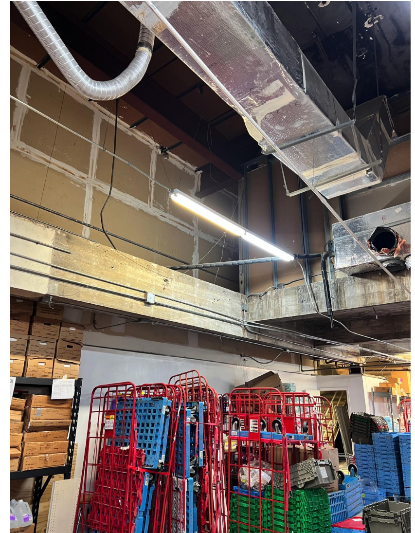
9. Storage Room at Ground Level
