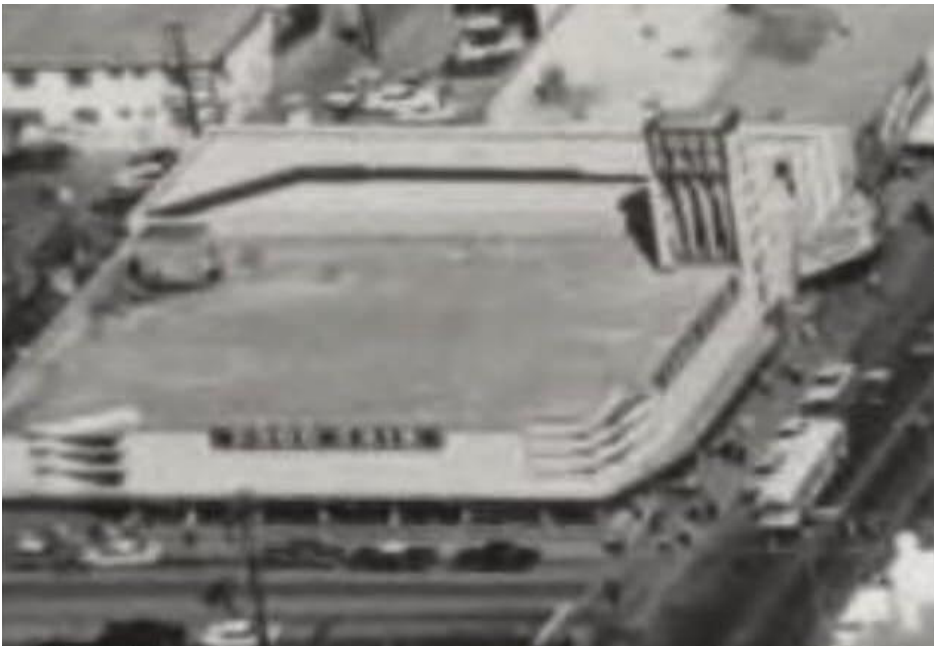
Aerial View of Food Fair Building 1950s
