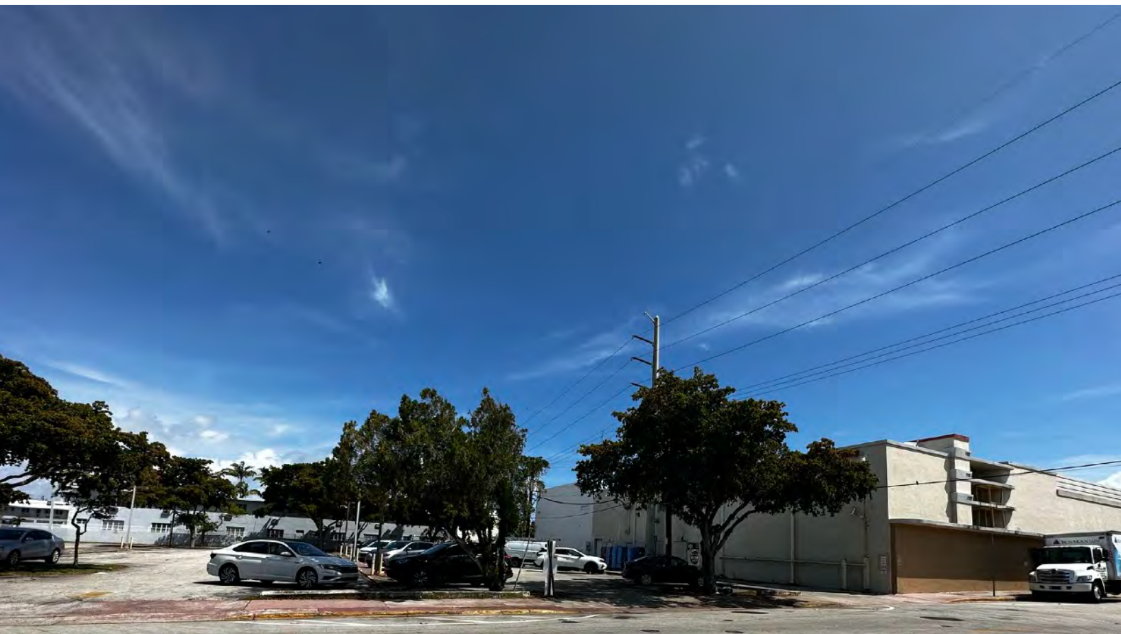
WEST ELEVATION WITH REAR PARKING LOT (11)
