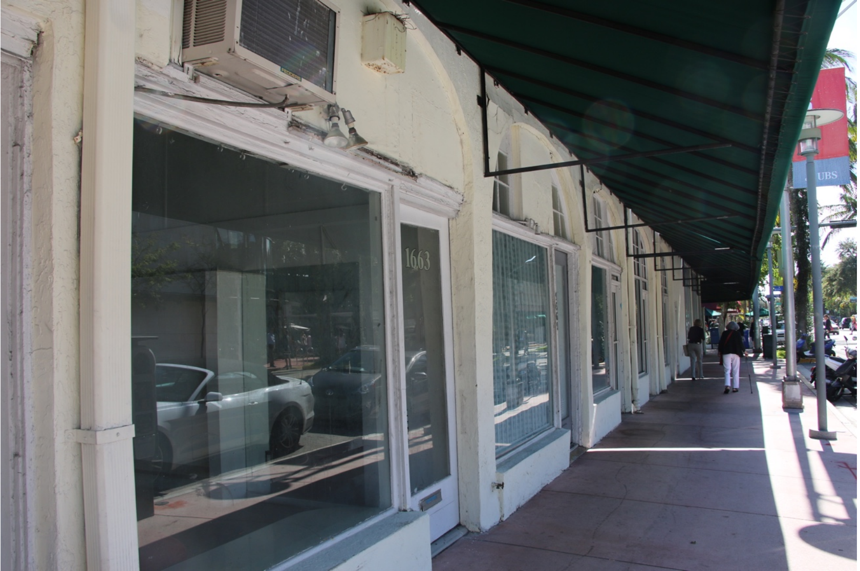
PHOTO ABOVE: VIEW SOUTH ALONG WEST ELEVATION
